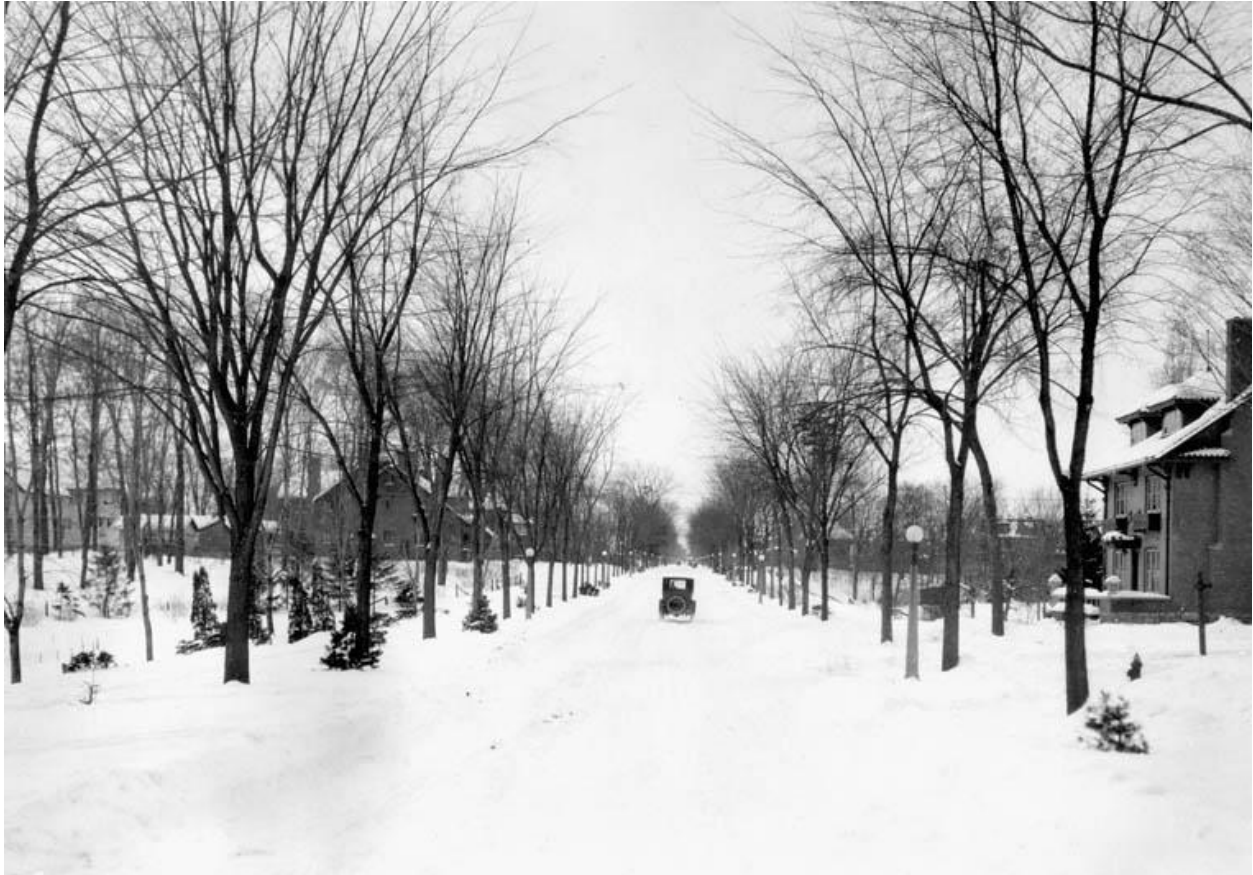
Figure 18: Monkland Avenue looking west, 1920s
