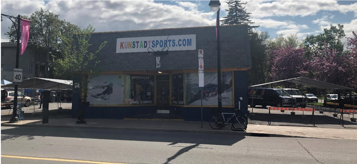
Figure 34: Commercial, non-contributing properties at 680 Bank Street
