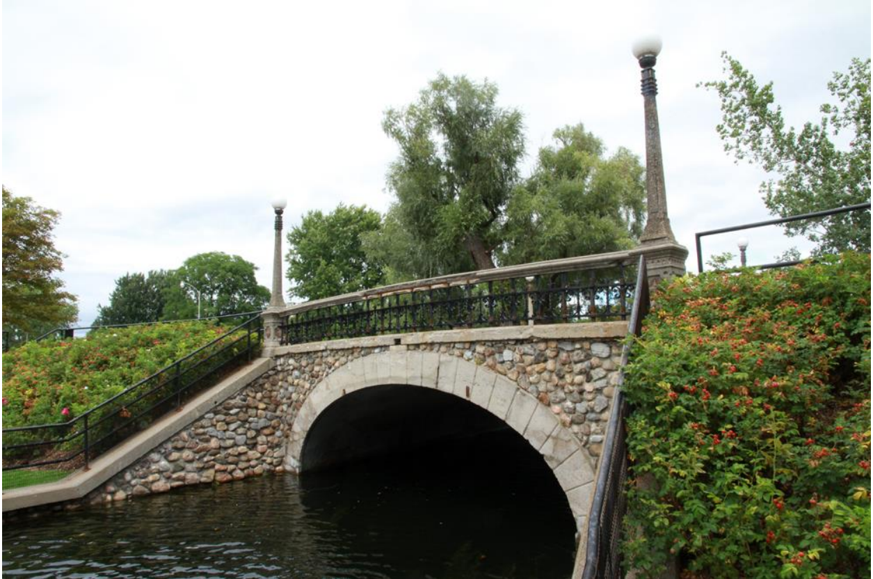
Figure 36: Patterson Creek Bridge
