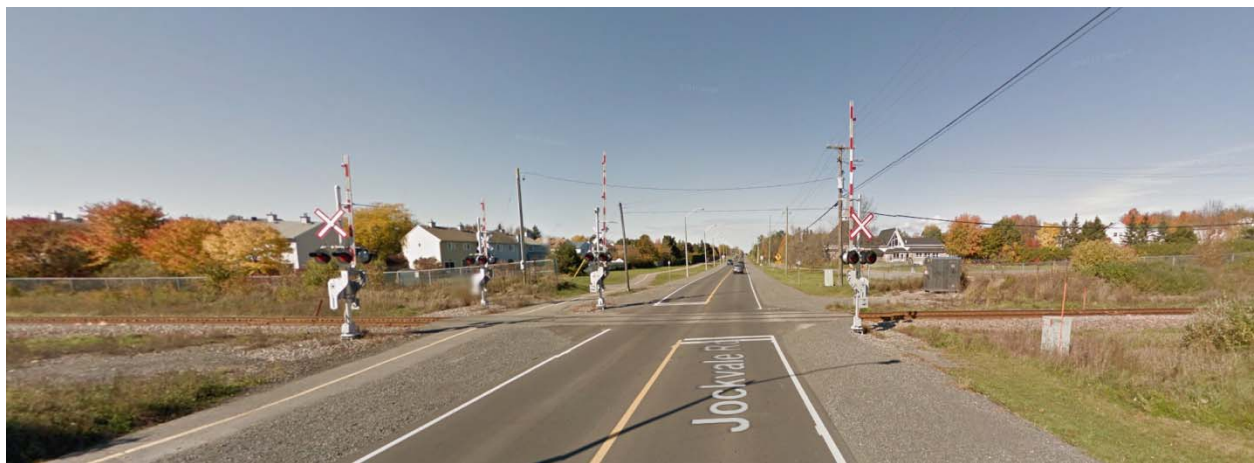
Figure 41: Street View Looking Northwest
