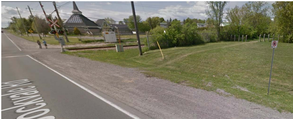
Figure 66: Current Pathway North of Jockvale Along Railway
