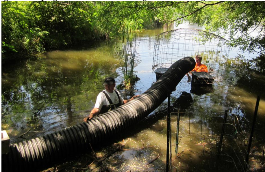
Figure A: Piping and round fence leading to culvert being installed
