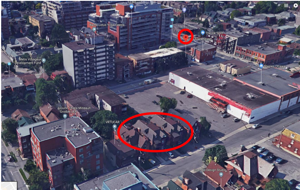
Figure 16: 3-D view of Frank Street looking south with the Staples parking lot in the middle of the image and the set of Category 1 and 2 houses on Waverley Street circled. Source: Google 3-D mapping with annotations by Contentworks.
