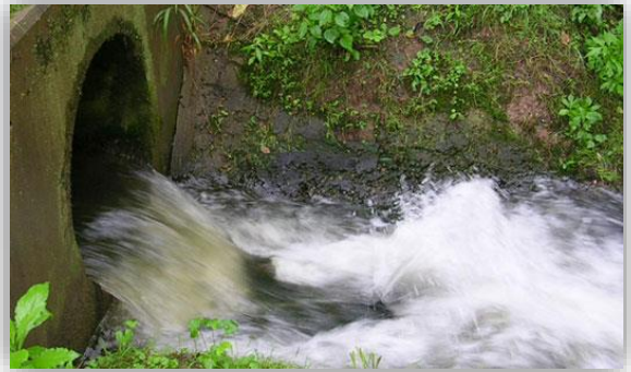
Storm Sewer Outlet
