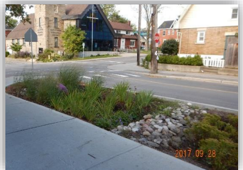
Example of Bioretention on Sunnyside Avenue, Ottawa (Conveyance Measure)
