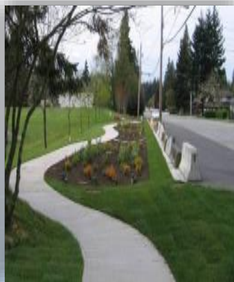
Bioretention/ Bioswales (Conveyance Measure)
