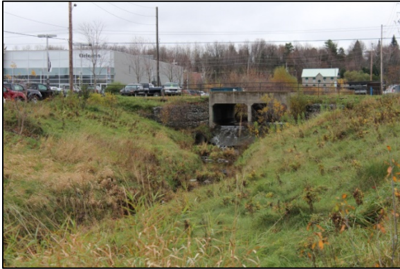
Photo 5: The Channelized Section of Voyageur Creek in the Youville Industrial Park
