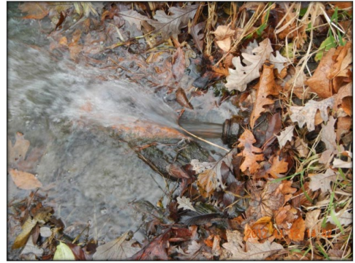
Photo 22: Erosion (Maintenance) site # 4 along Reach VC-1
