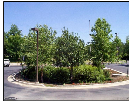
Photo 37: Bioretention Unit in a Cul-de-Sac
