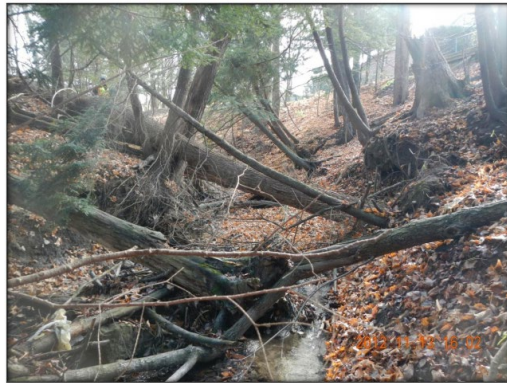
Photo 25: Erosion site #5 along Reach VC-5
