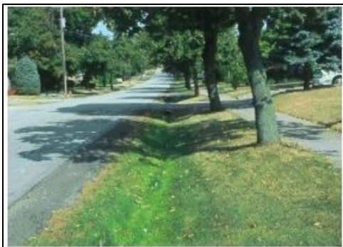
Photo 40: Grassed Swales Infiltrate Stormwater and Improve Water Quality
