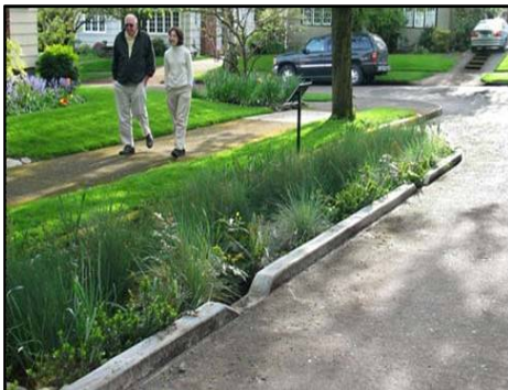
Photo 36: Bioretention Unit Along the Road
