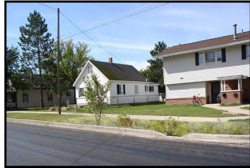
Photo 35: Completed Bioretention Unit in the Road Boulevard
