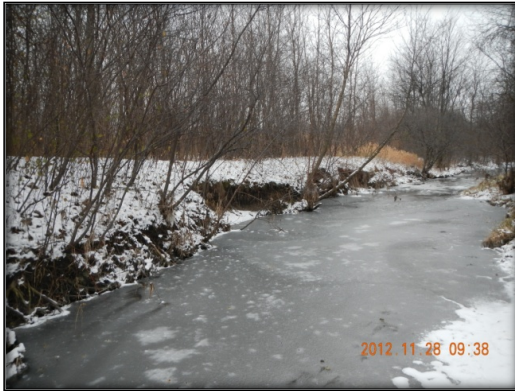
Photo 15: Typical Erosion Conditions Identified Along Cyrville Drain Consisting Of Steep Banks And Exposed Roots.
