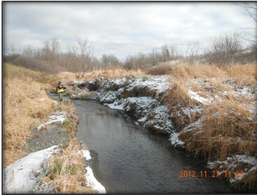
Photo 19: Typical Erosion Conditions Along McEwan Creek Consisting Of Slumped Bank Material.
