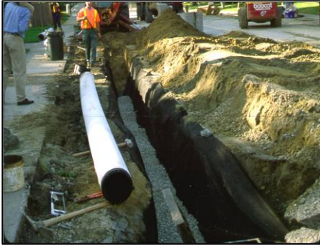
Photo 38: Exfiltration Trench / Perforated Pipe System During Construction
