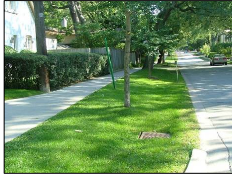
Photo 39: Exfiltration Trench / Perforated Pipe System After Construction
