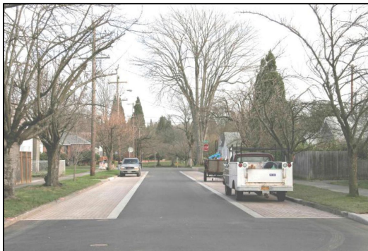
Photo 41: Permeable Pavement Use within the Municipal Right Of Way
