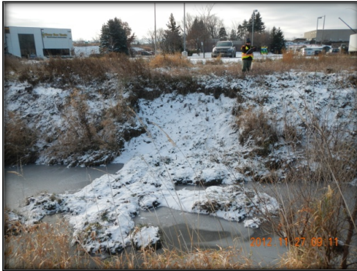
Photo 17: Typical Erosion Conditions Along Mather Award Drain Consisting Of Slumped Bank Material.
