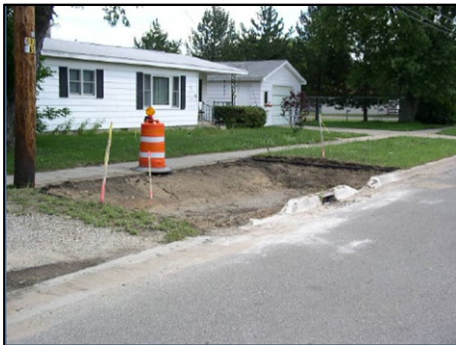
Photo 34: Bioretention Unit During Construction
