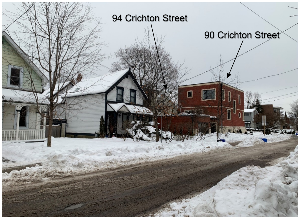
View of rear of 90 Crichton Street (right) and roofline and rear façade of 94 Crichton Street (immediately left) shown from Queen Victoria Street.
