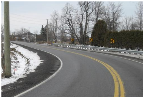
Figure 24 - Guiderail along a curved road
