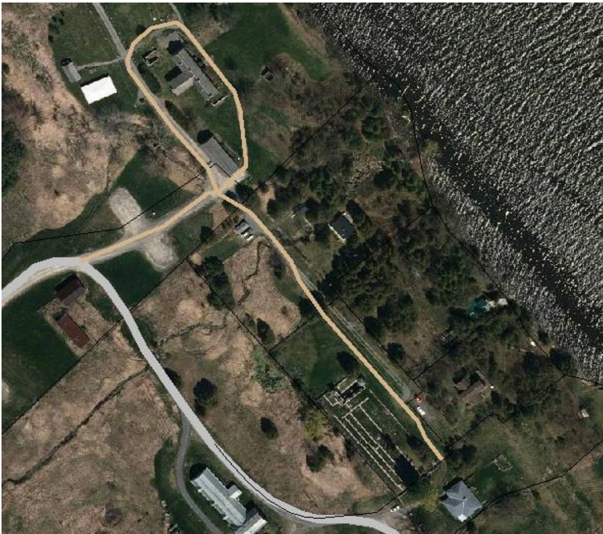
Aerial view showing relationship of Old St. Mary's to Horaceville (City of Ottawa)
