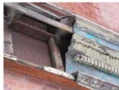
Low Level Cornice to be Replicated
