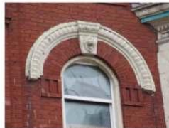
Arched Window Metal Work Details to be Restored
