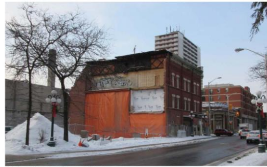
Existing structure at Somerset Street
