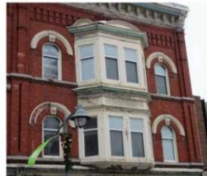
Existing Bay Window Structure to be Reconstructed
