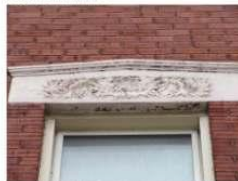
Precast Stone Window Headers to be Restored
