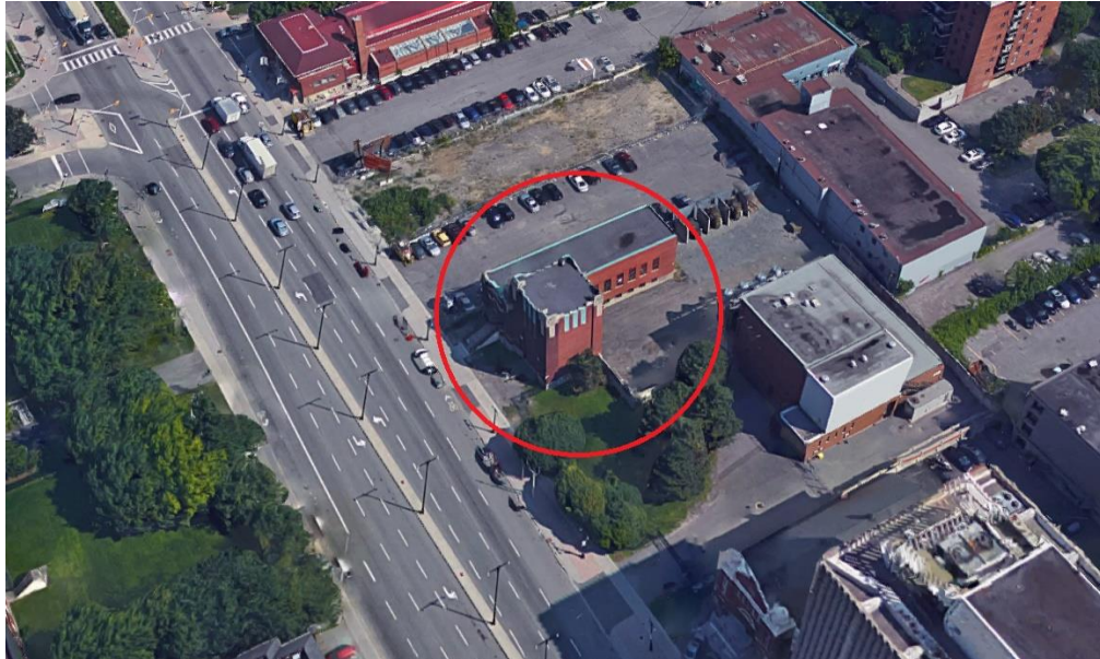
Photo showing Hydro Sub-Station No. 4. Source: © 2019 Google
