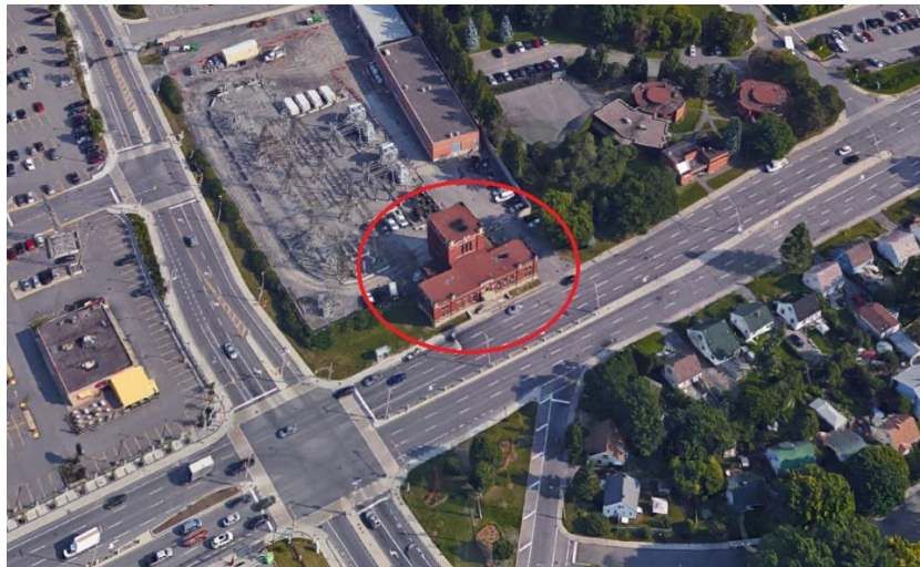
Photo showing Hydro Sub-Station No. 3. Source: © 2019 Google.
