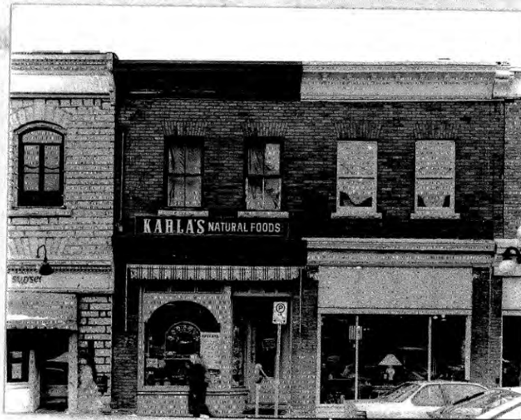
Attach building photos here: 1 - 6 x 6
