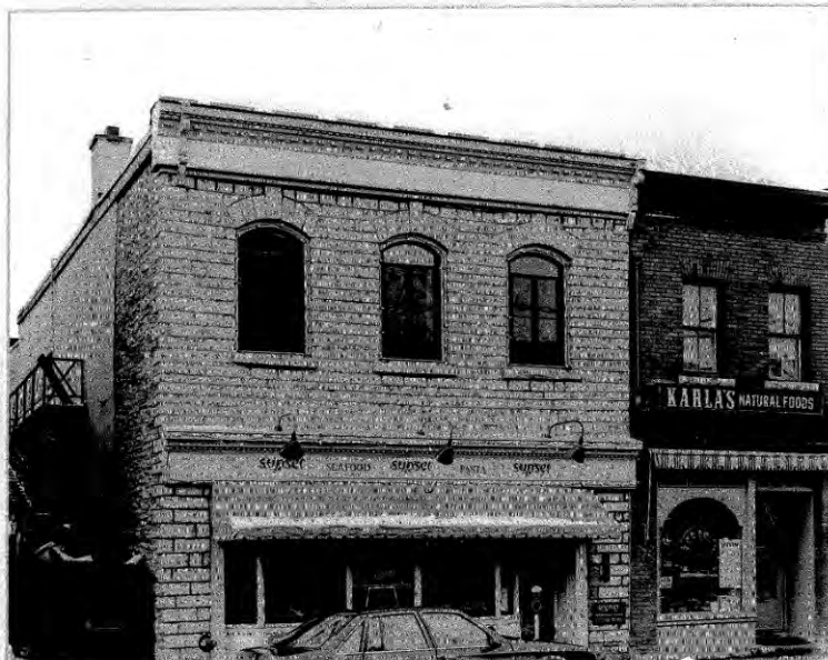
Attach building photos here: 1 - 6 x 6
