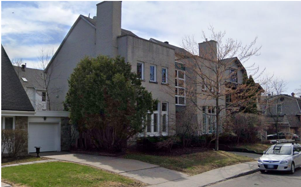
Figure 11: 115-117 MacKay Avenue viewed from the street, the two-storey split double with shared driveway is a handsome expression. The flat roof with side gables is a contemporary version of this traditional form and provided a model for the previous scheme. Source: Google Earth
