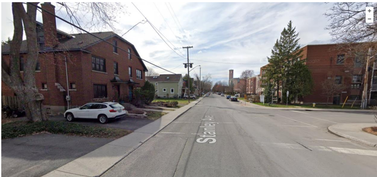
Figure 6: View looking north at the intersection of Keffer Avenue. The three-storey apartment at the opposite side of the street 174 Stanley Avenue is a conversion from the City Archives, which was a conversion from the Ste. Vincent School. The semi is approximately the same height as the apartment. Source: Google Earth.
