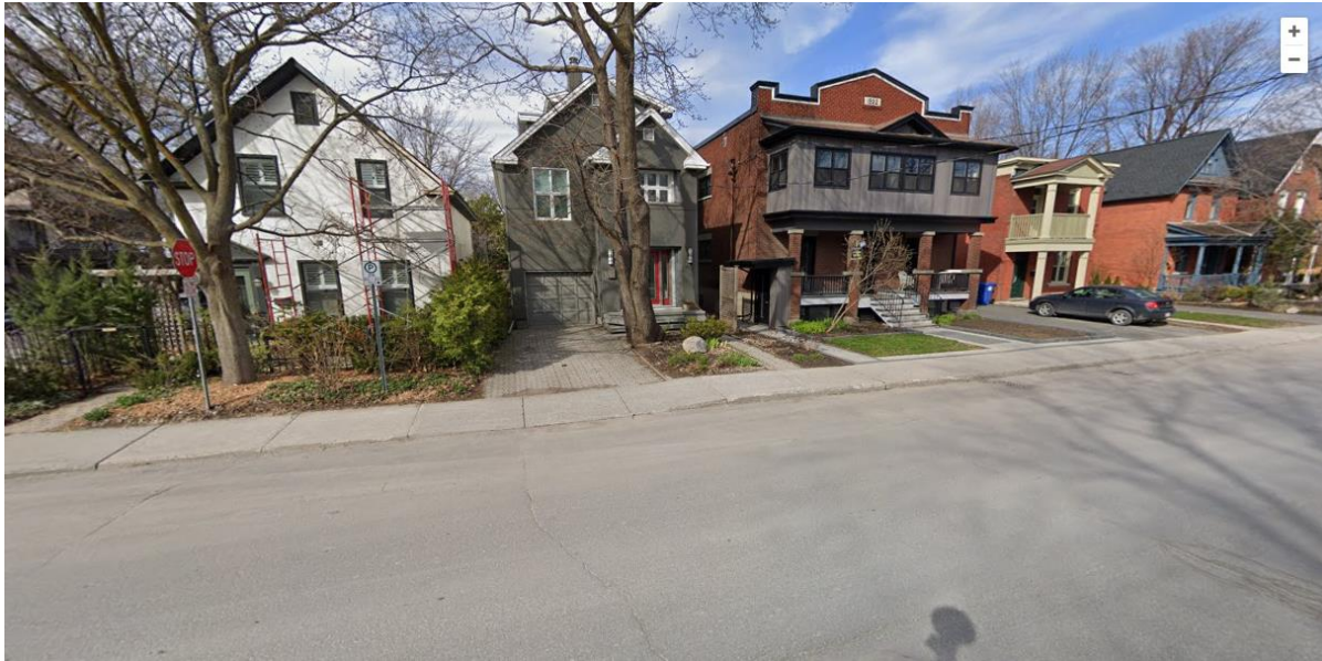
Figure 7: View of residences on the east side of Stanley Avenue. 10 Keefer appears on the 1912 fire insurance map as a double lot with 188 Stanley address. After 1912, the lot was severed to form three properties 10 Keefer, 188 and 190 Stanley Avenue. The boomtown front at 190 Stanley with a flat roof is c.1920. The closed in upper floor porch adds character and bulk to the front façade. The flat roof at 192, and the twinned end gables at 194-and196 Stanley Avenue, appear on the 1901 /1912 revised FIP. Source Google Earth
