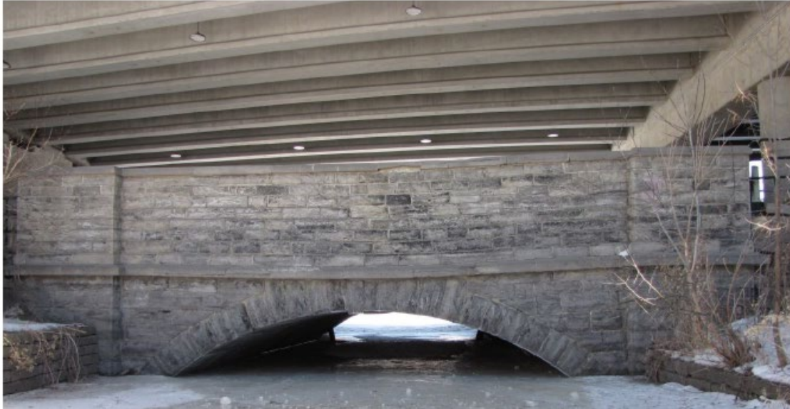
West façade, Booth Street Bridge
