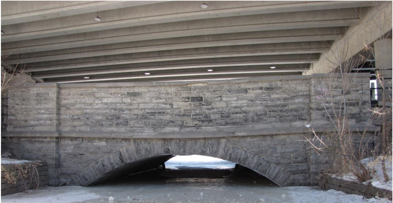
Figure 1: West arch and parapet of the Old Booth Street Bridge, March 2019. Source: Parsons.
