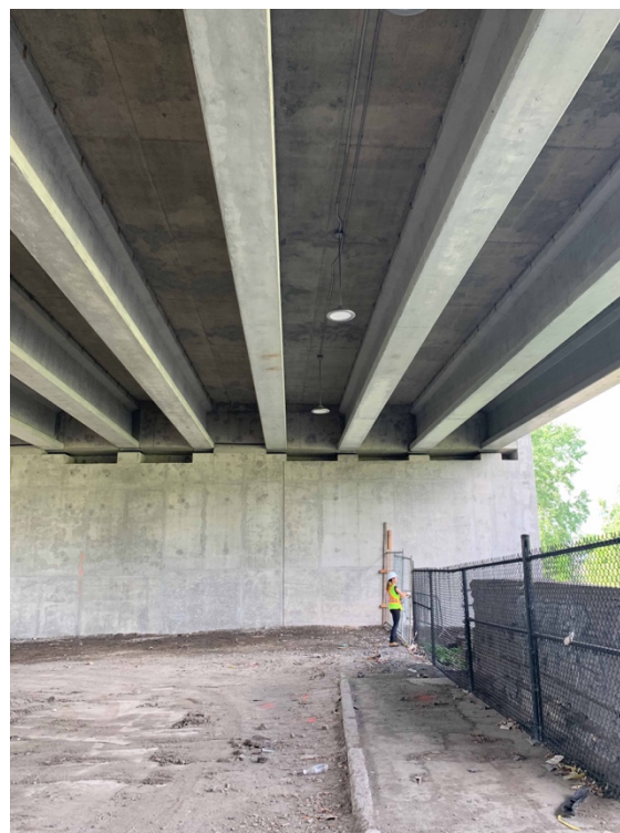
Figure 7: Photo of the Old Booth Street Bridge looking north towards the concrete wall abutment supporting the overhead Booth Street Bridge, 2019.
