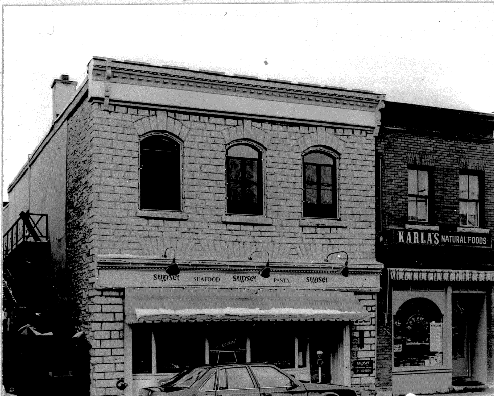
Attach building photos here: 1 - 6 x 6
