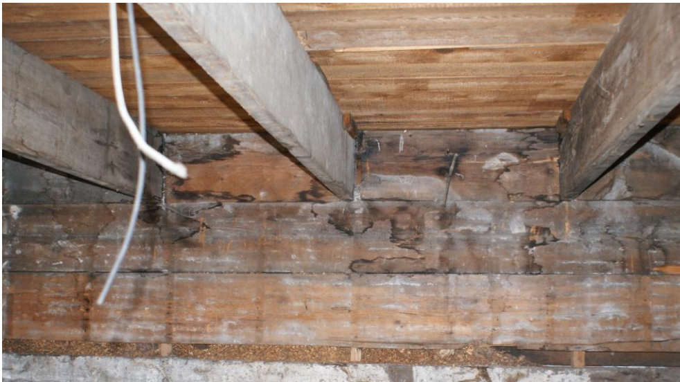
Figure 4: View of the balloon frame construction with second floor joists in the rear wing supported on 2" x 4" studs which are visible at the bottom of the photograph.
