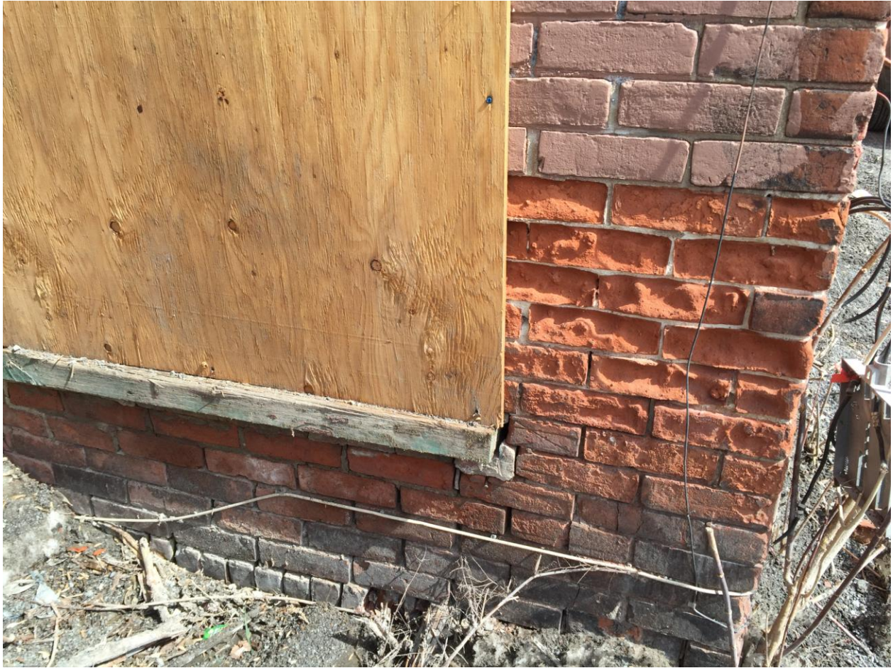
Figure 14: View of the deteriorated brickwork and pointing. Credit: Neil Zaret 2016.
