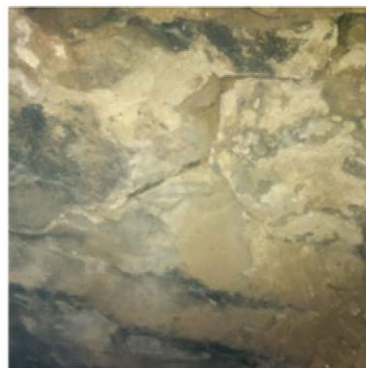
Photo Four – Deteriorated Mortar
