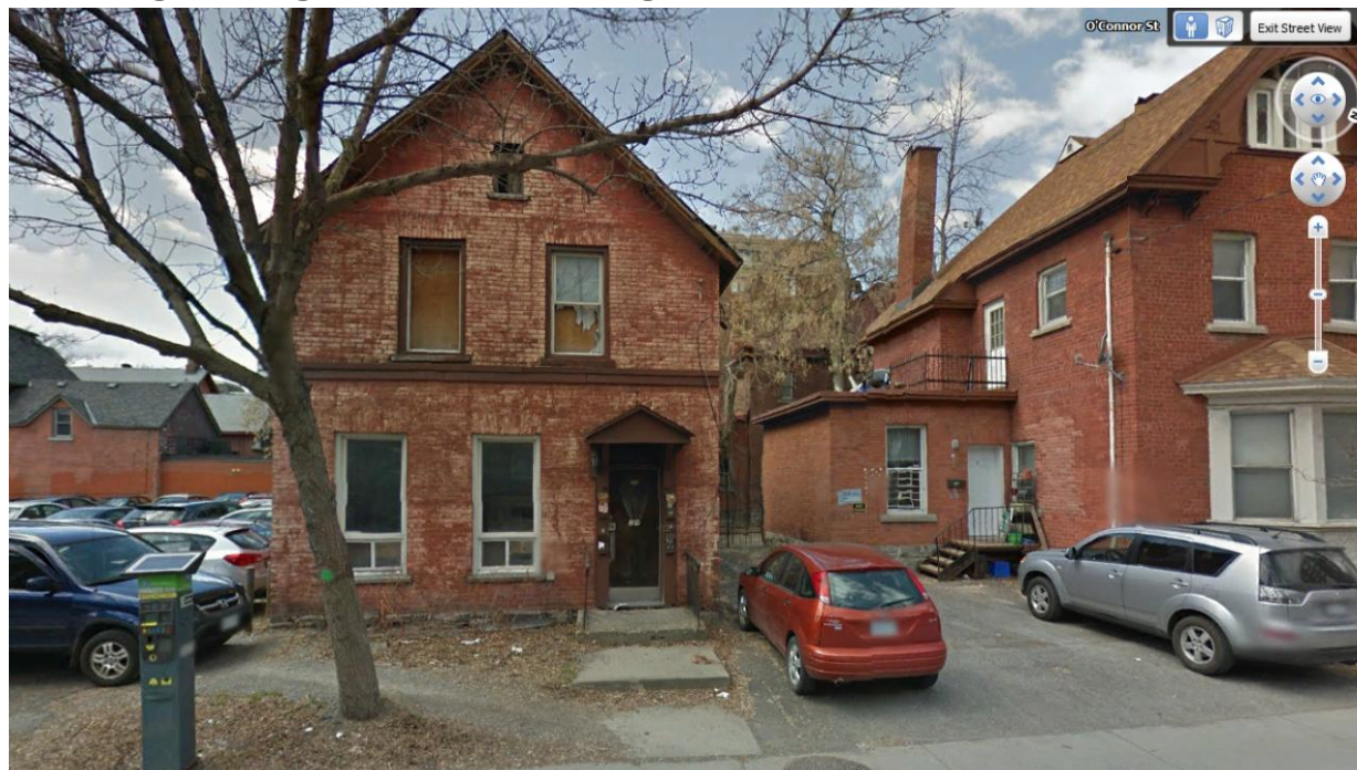
Figure 8: Context view of the site at 234 (left) O'Connor Street. The building is identified as Category 2 heritage resources in the HCD Plan. The exterior brick was painted to protect the relatively soft brick and has peeled off due to the building being vacant and unheated. Credit: Google Earth 2015
