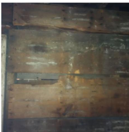
Photo Two – Dry Rot on Wood Framing
