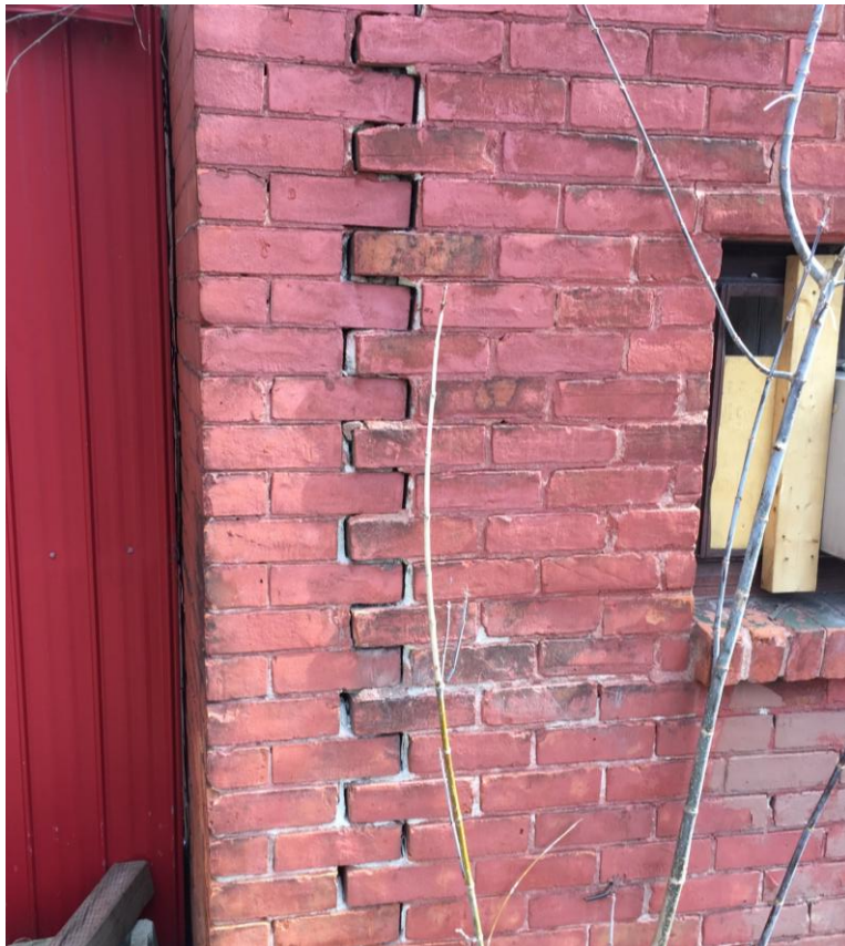
Figure 8: View of the west wall of rear wing illustrating the detached brick veneer.
