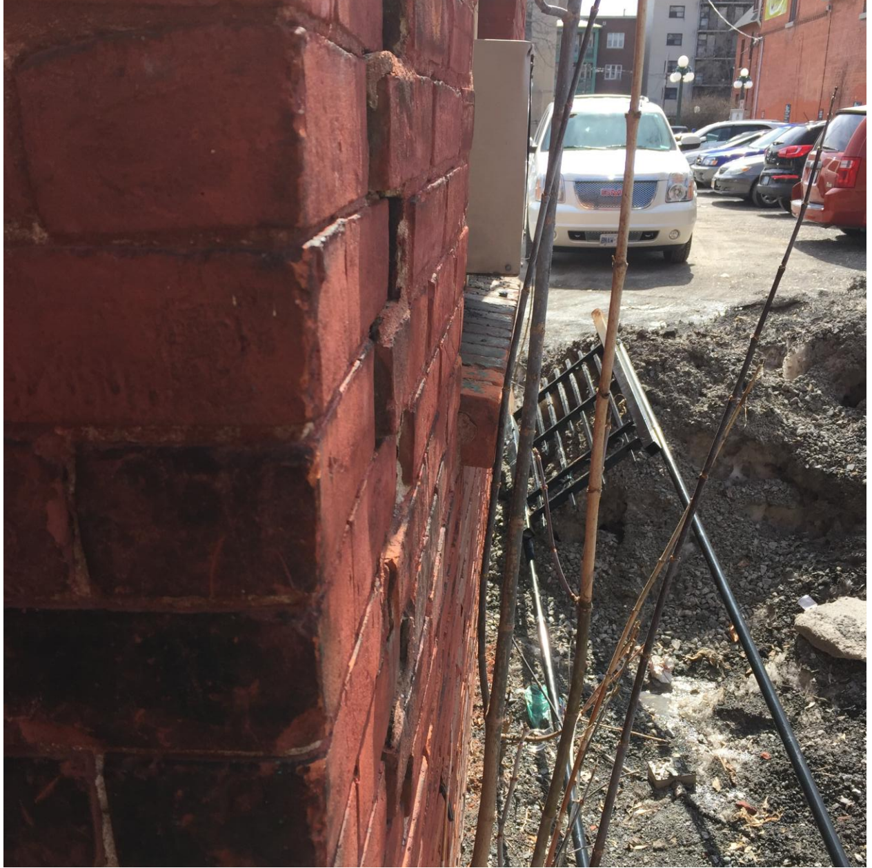
Figure 12: View of the rear (west) wall showing the outward displacement of the brick veneer. Credit: Neil Zaret 2016.
