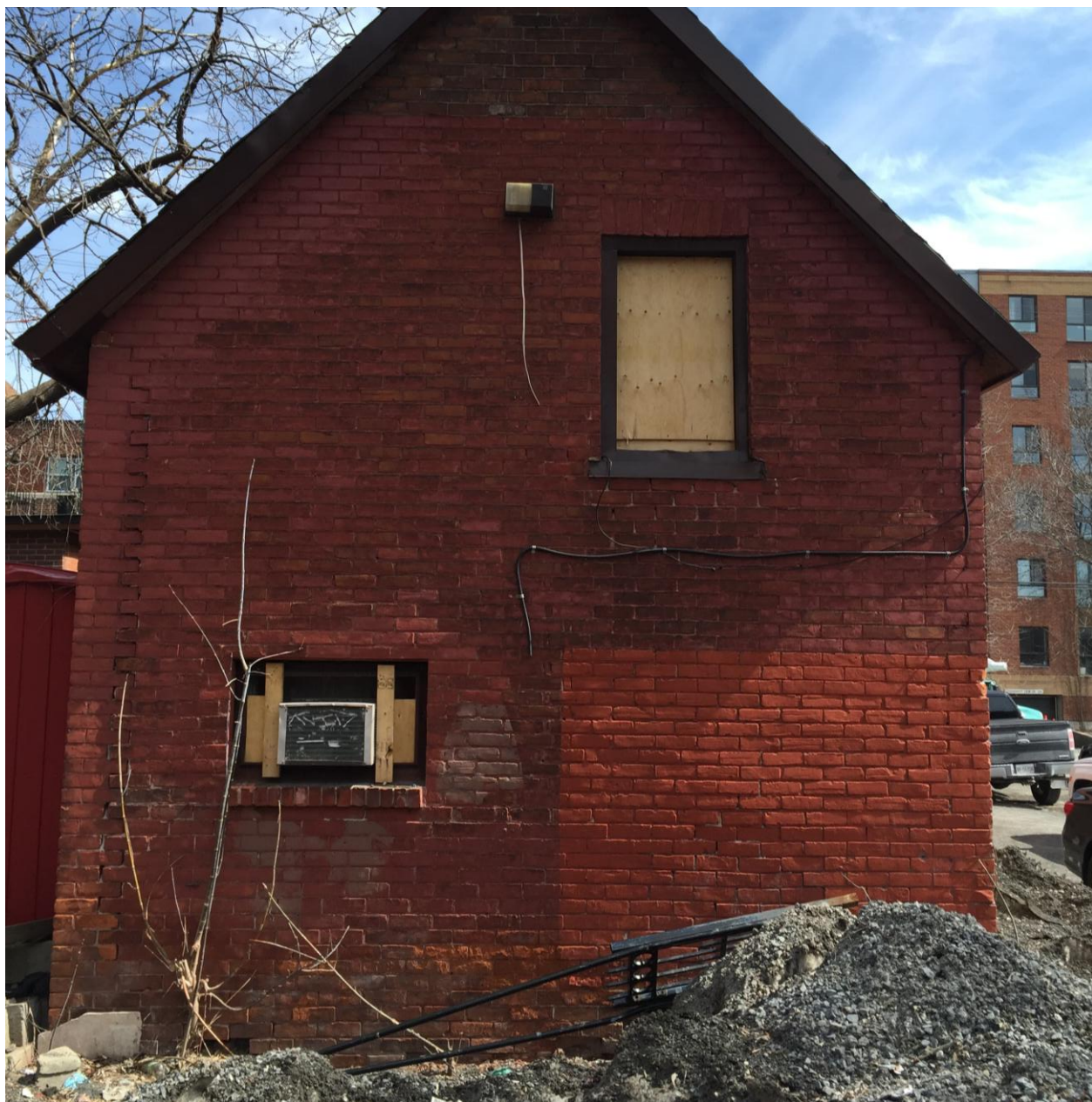
Figure 10: View of the rear (west) wall of the building. Note the structural crack in the brick veneer extending up the left corner of the building due to settlement / movement in the stone foundation. Credit: Neil Zaret 2016
