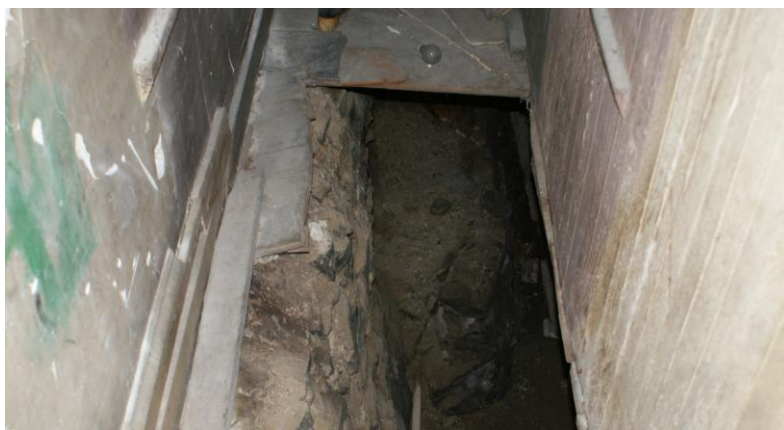
Figure 5: View down the stair to the basement. Note the displaced foundation wall which has been pushed into the building and the floor boards which have rotated upward.
