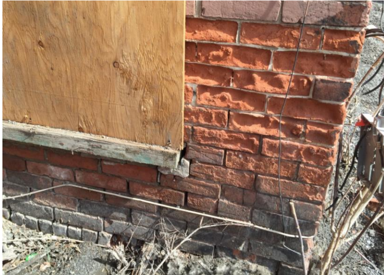
Figure 7: View of deteriorated brick at the base of the wall at the south-west corner of the front half of the building. Note the raised grade above the level of the stone foundation, and the buried brick headers at the top of a basement window.
