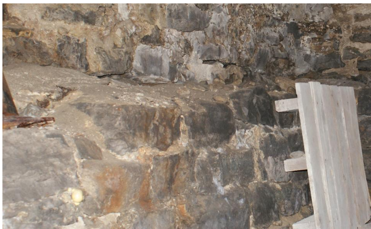
Figure 6: View of the foundation wall in the basement. Note the secondary stone wall at the base of the upper wall. This is a typical condition for foundation walls in front half of the building.
