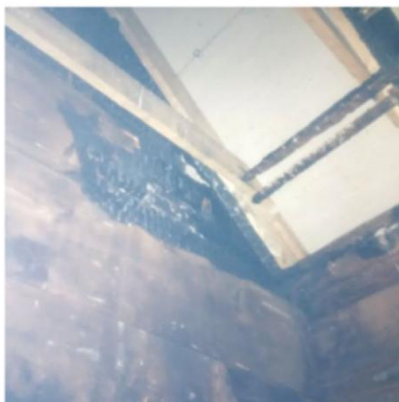
Photo One – Fire Damaged Roof Framing
