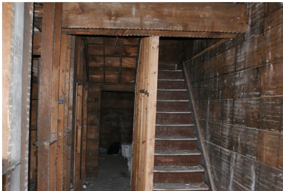
Figure 2: View of the interior stair. Note the horizontal board sheathing applied to the interior walls.
