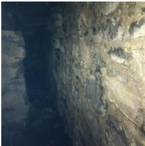
Photo Three – Rubble Stone Wall
