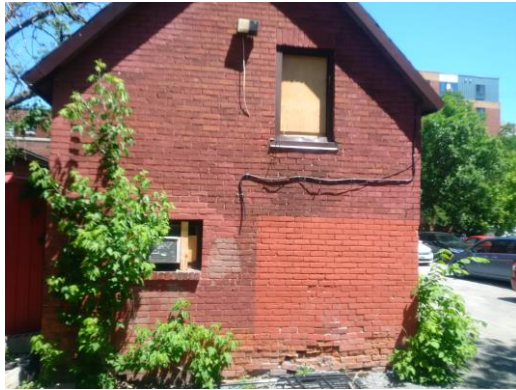
Photo Five – West Elevation Brick
