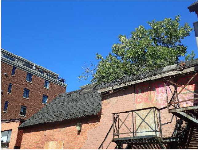
Photograph 8 – Roof of rear additions, JCAL (2016)
