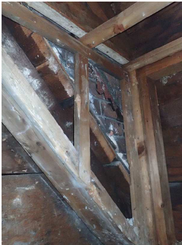
Photograph 4 – Brick supported on wood framing, JCAL (2016)
