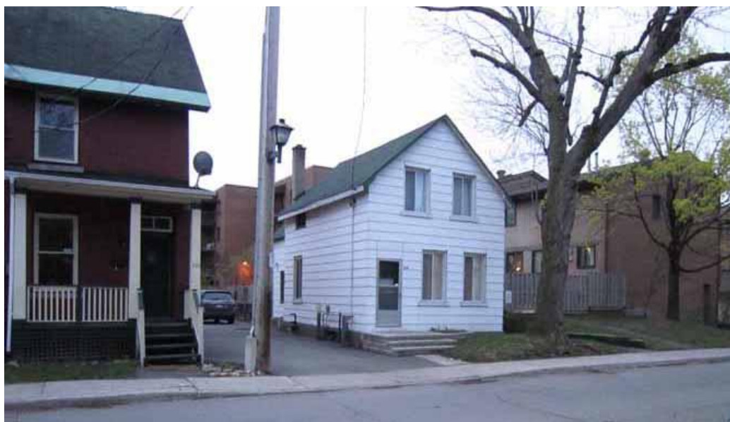
Figure 4: 216 Cathcart St (white house) flanked by house c. 1900 on left and infill multi-unit housing c. 1980 on right. Source: Contentworks, 2012.
