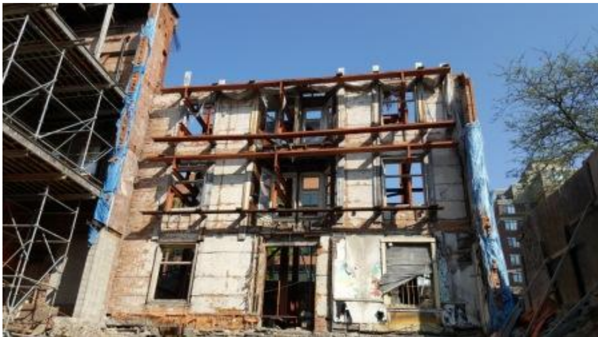
Interior wall, Easterly bays, site of complete demolition (GL 5-8).
