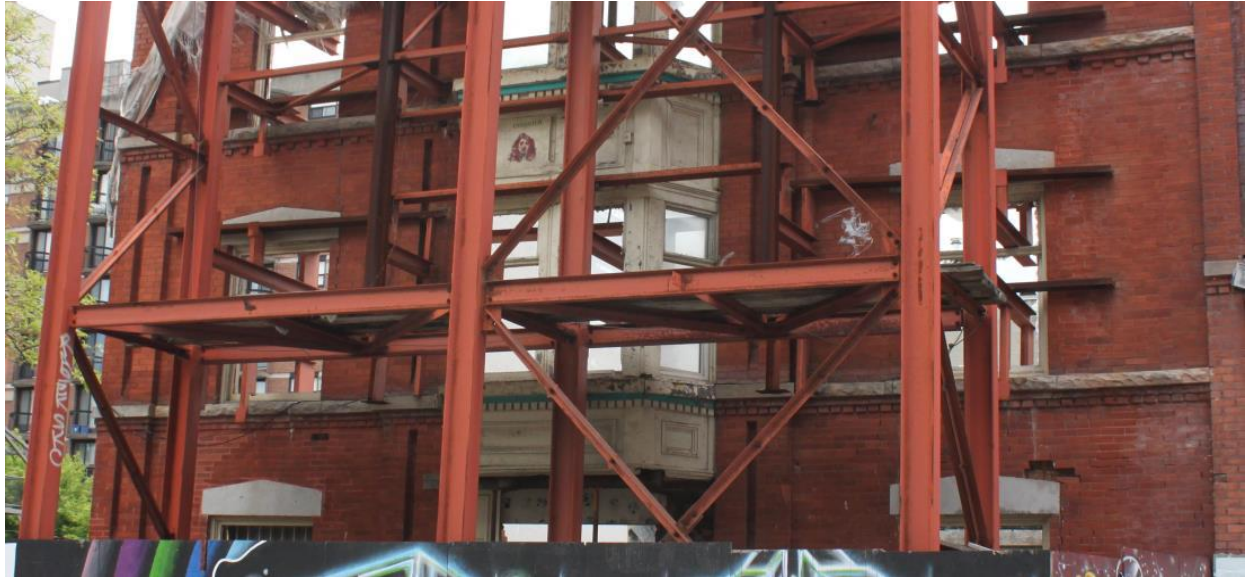
Exterior Wall, Easterly bays, site of complete demolition (GL 5-8)
