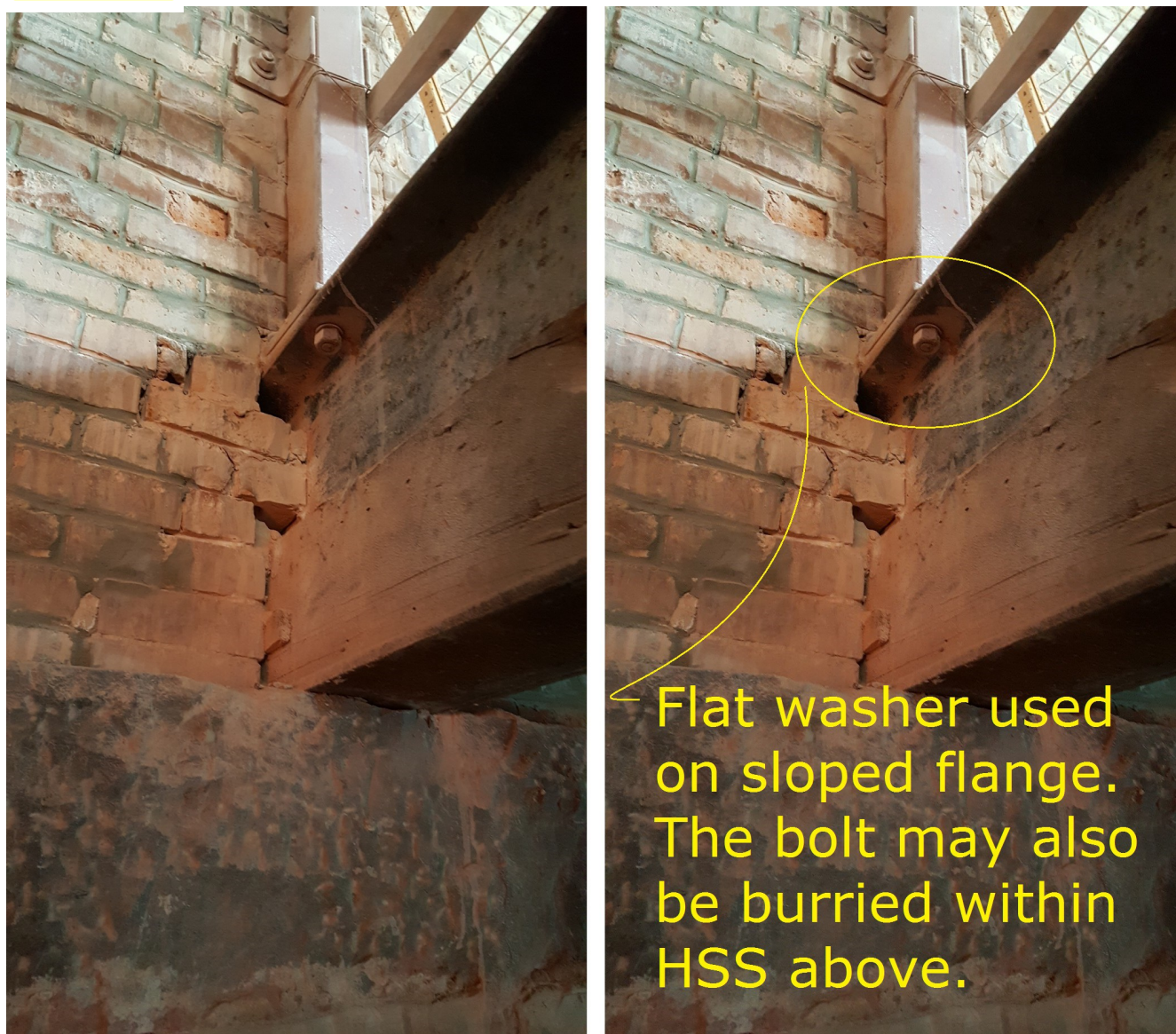
Photo 4.1 - Flat washer and resultant twisted bolt on S shape
