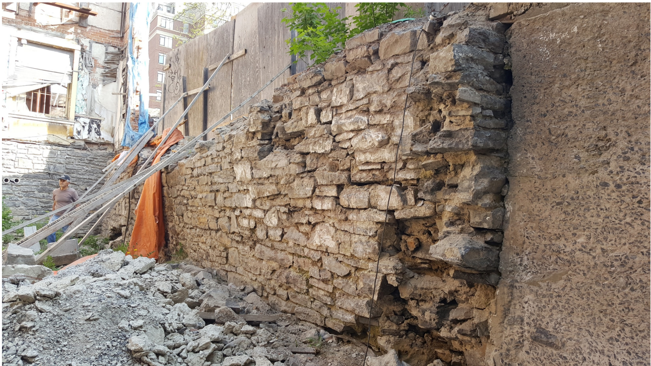
Photo 1.3 - Failing Stone Foundation at adjacent Parking Lot
