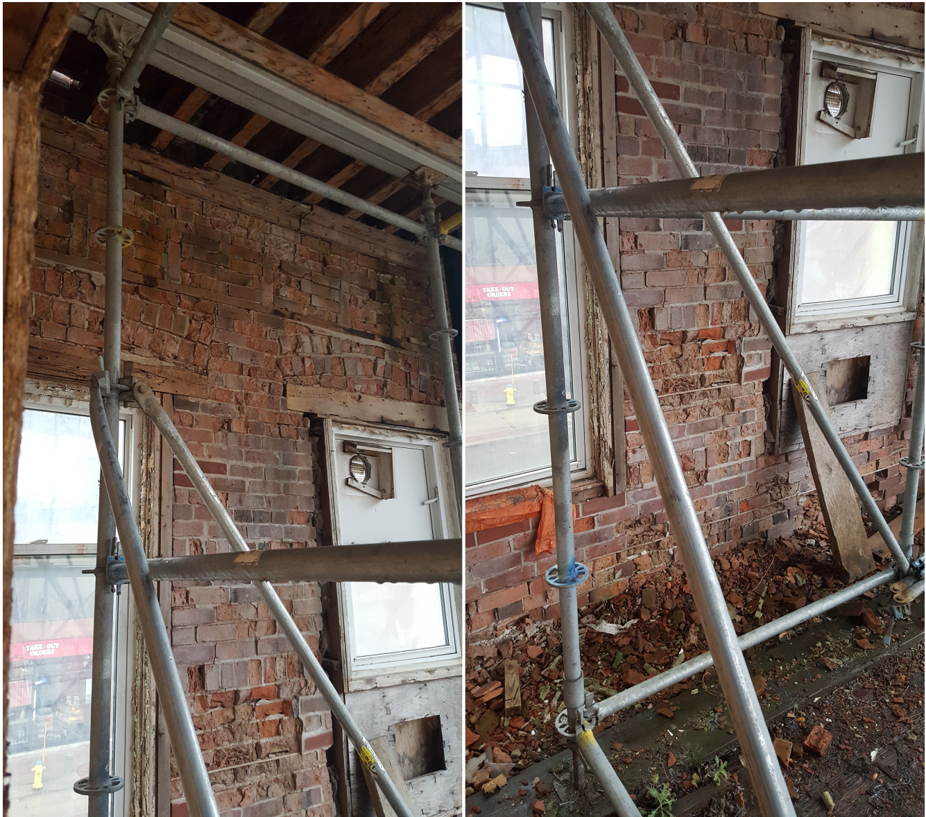
Photo 1.4 - Masonry Wall Deterioration along GL A from GL 4 to 5
