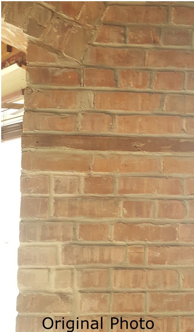
Photo 3.2 - Segmental Arch Abutment Cracking
