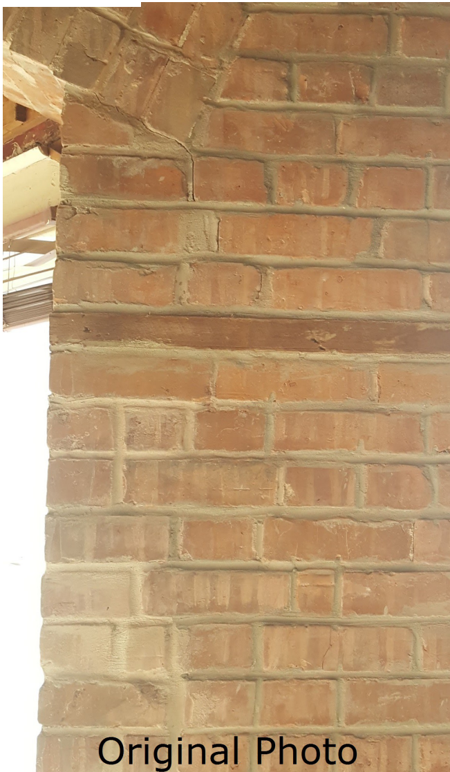
Photo 3.2 - Segmental Arch Abutment Cracking
