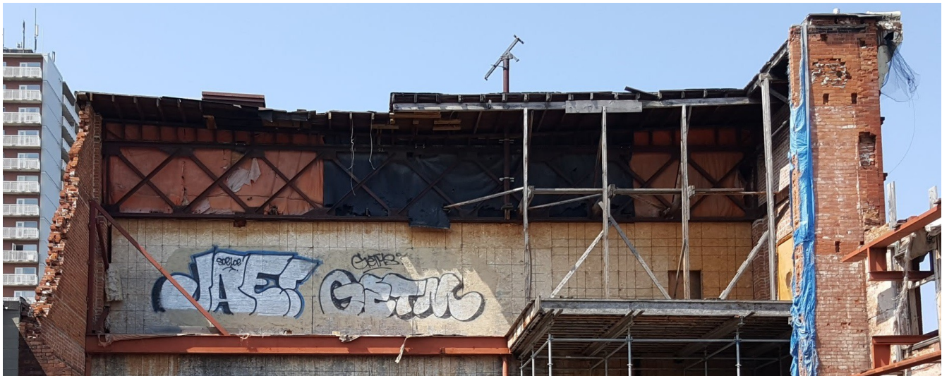
Photo 3.1 - Heritage Roof Truss Exposed to Elements
