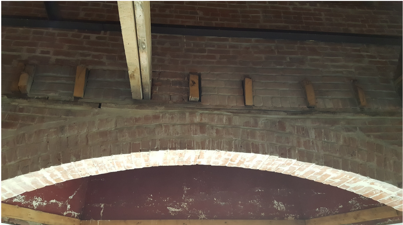
Photo 2.1 - Cut off Ceiling Joists
