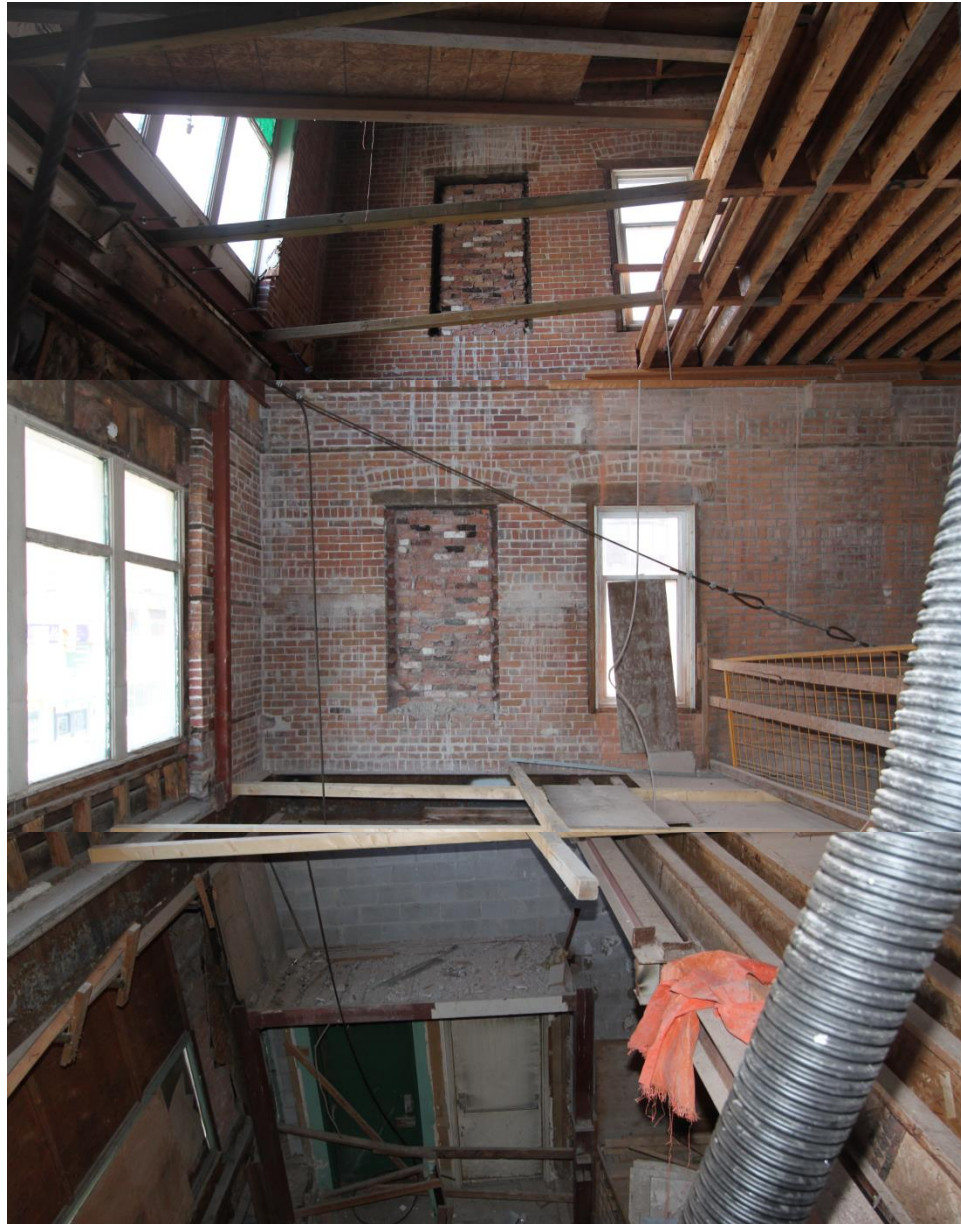
Figure 8. Composite view of the unsupported walls at the corner of Bank and Somerset Streets
