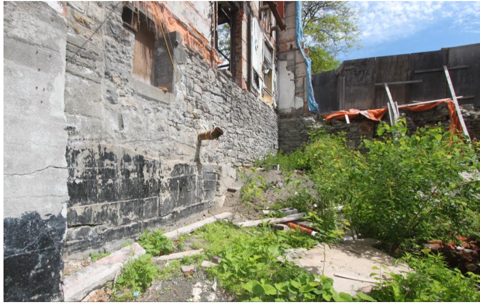
Figure 4. View of the part of the Somerset Street façade foundation wall and the partly collapsed foundation along the parking lot in the background
