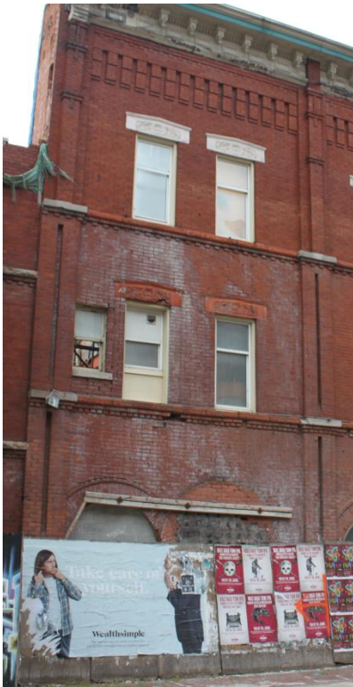
Figure 6. Efflorescence as evidence of constant wetting of the wall
