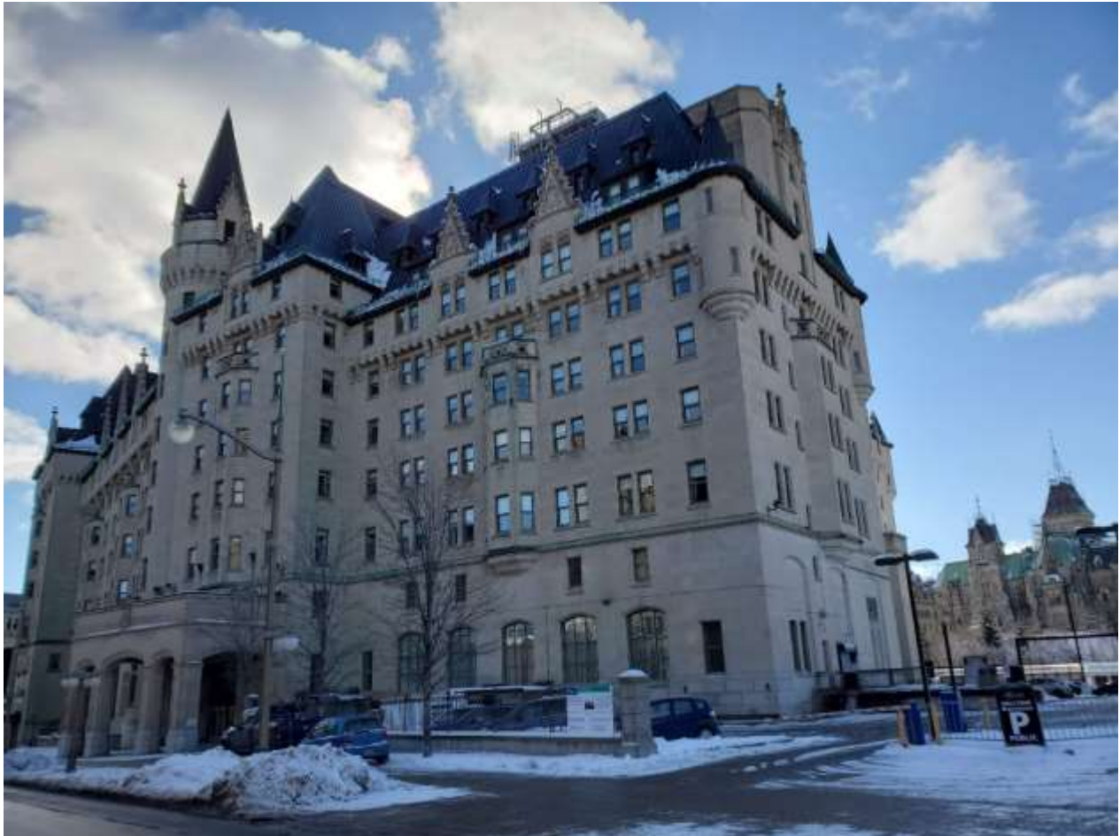
Façade est, avenue Mackenzie
