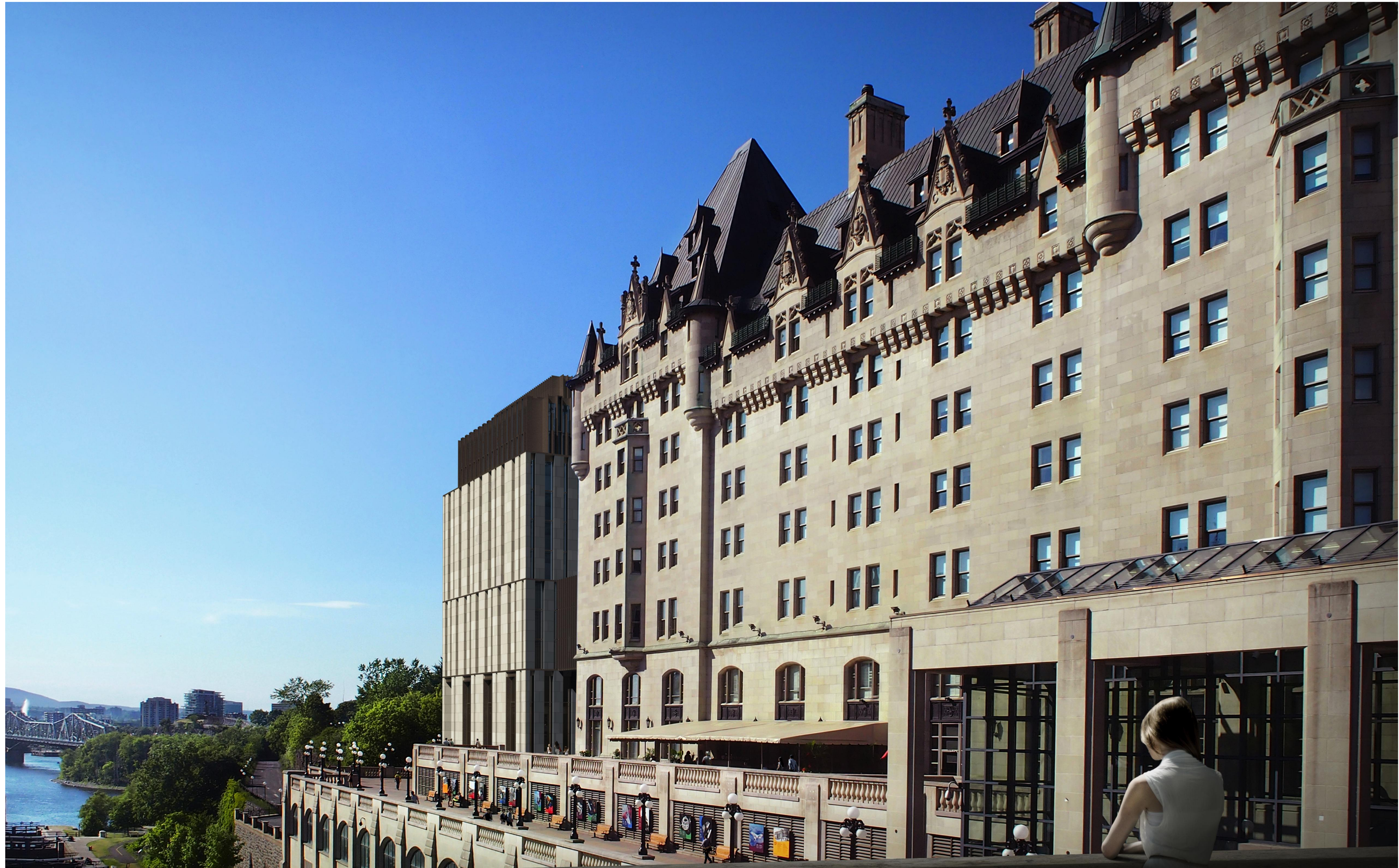
VIEW FROM THE WELLINGTON STREET BRIDGE
