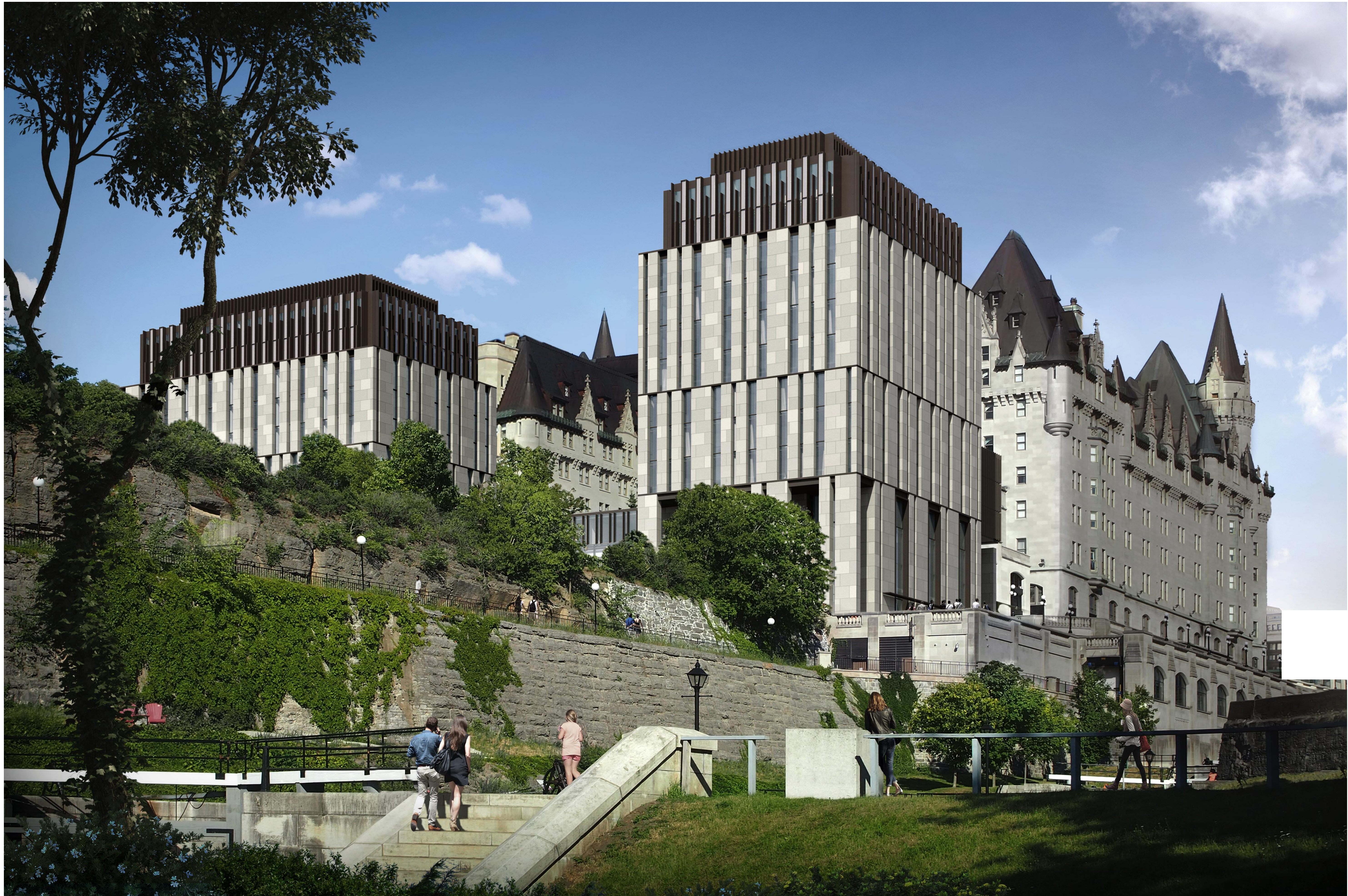
VIEW FROM THE RIDEAU CANAL LOCKS
