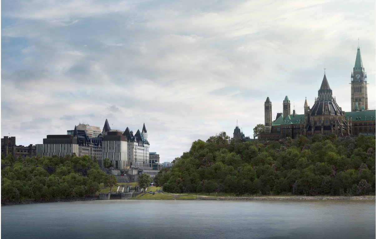
23. View analysis of the proposed addition, looking south from the Ottawa River (Source: architectsAlliance)
