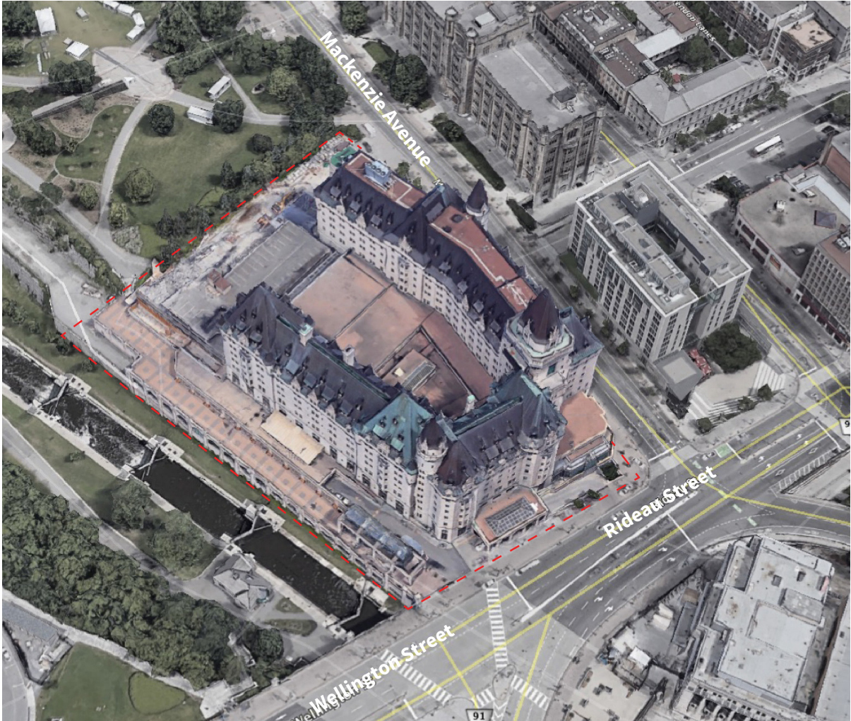
1. Axonometric view of the Development Site, outlined in red (Source: Google Maps, annotated by ERA).
