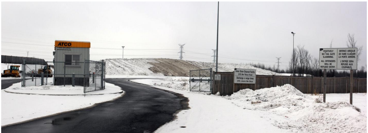
Figure 3. Snow Disposal Facility
