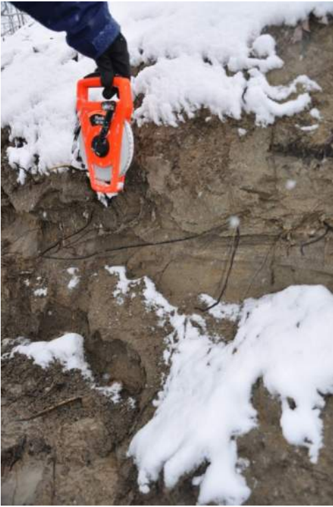
Photograph 5 ↑ Close up of side wall in groundwater fed channel. Note the 1m thick layer of fine sand over clay.
