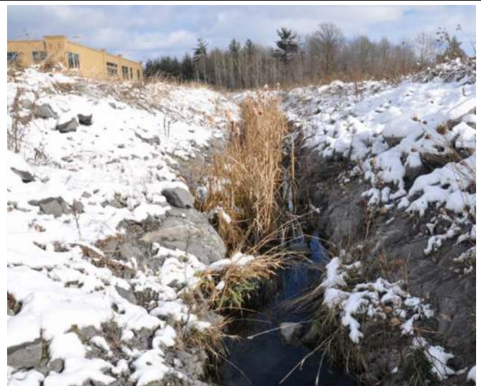
Photograph 4 ↑ Lindsay Formation Bedrock within the drainage channel leading into the Interim SWM Pond.
