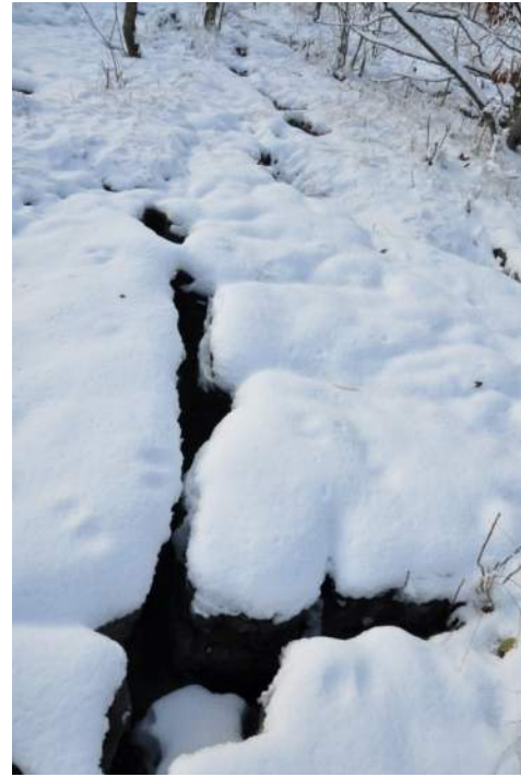
Photograph 2 ↑ Lindsay Formation Bedrock. Solution enhanced fracture.
