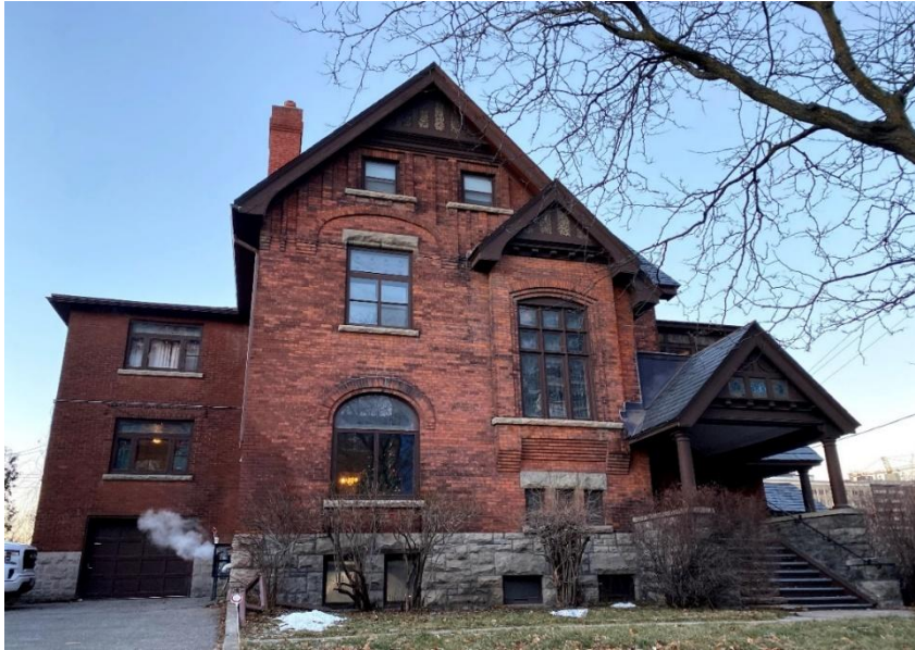
593 Laurier Avenue West, Alexander Fleck House, south façade.
