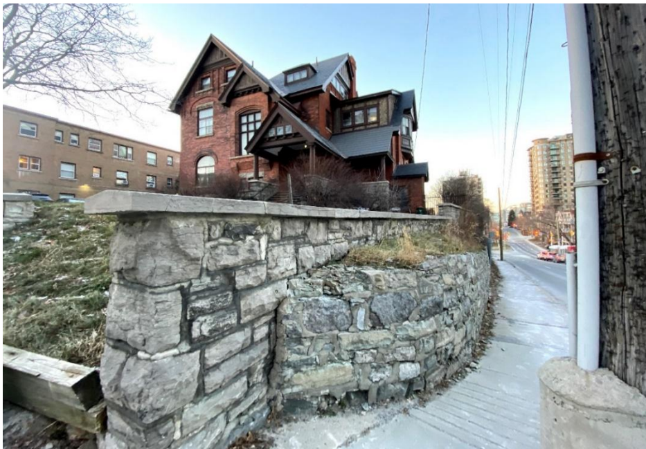
Photo from the corner of Bronson and Laurier Avenues, showing the stone wall along the edge of the property.
