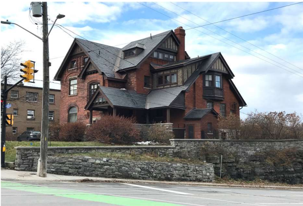
Figure 9: 593 Laurier Avenue, side (south-west) façade of existing building. (RMA)
