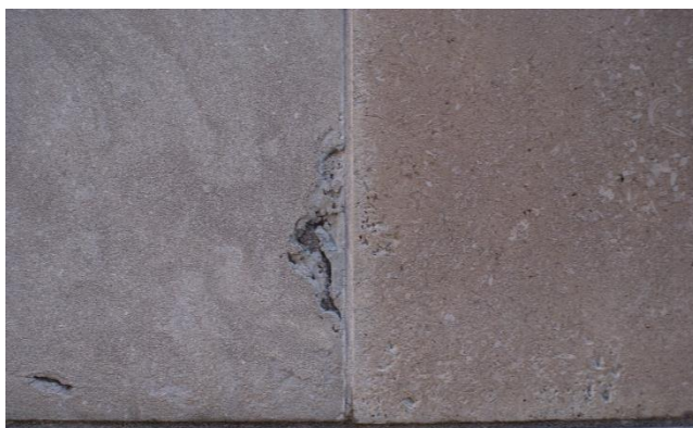
Figure 8: Detail view of ashlar limestone blocks with voids or vugs in the unit to the left. Note the shell fossils in the block to the left. Source: CHRM.
