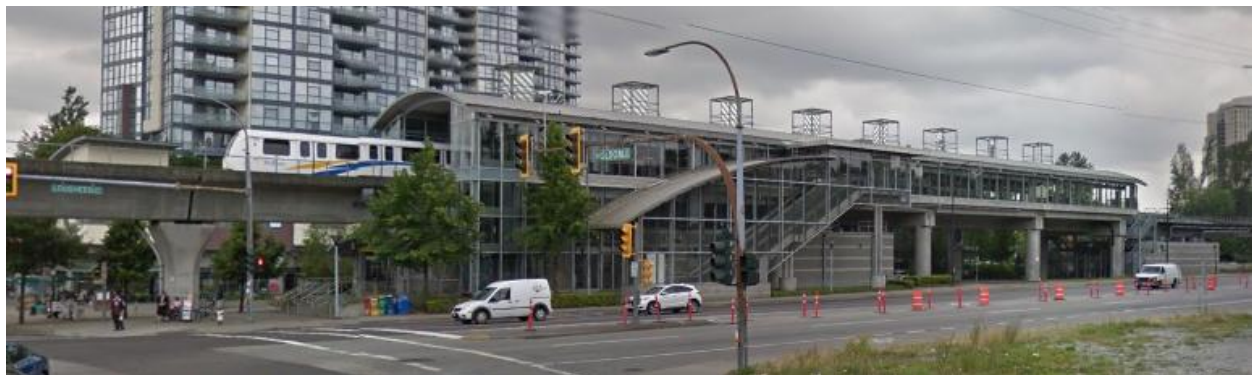
Figure 16: Vancouver Skytrain Example of Elevated Station
