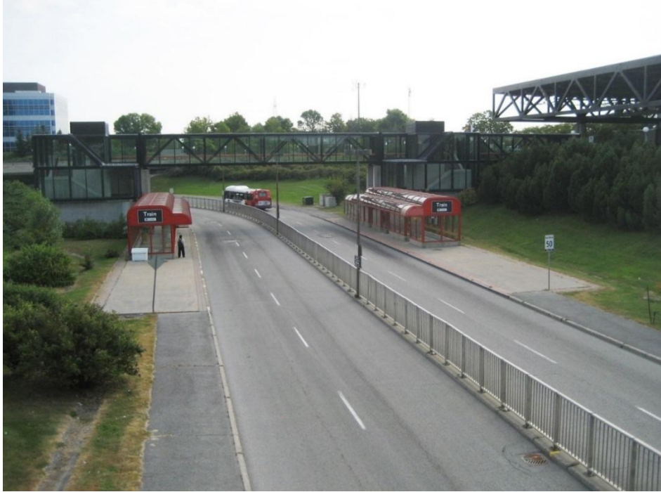
Figure 17: Fully Segregated BRT (Ottawa)
