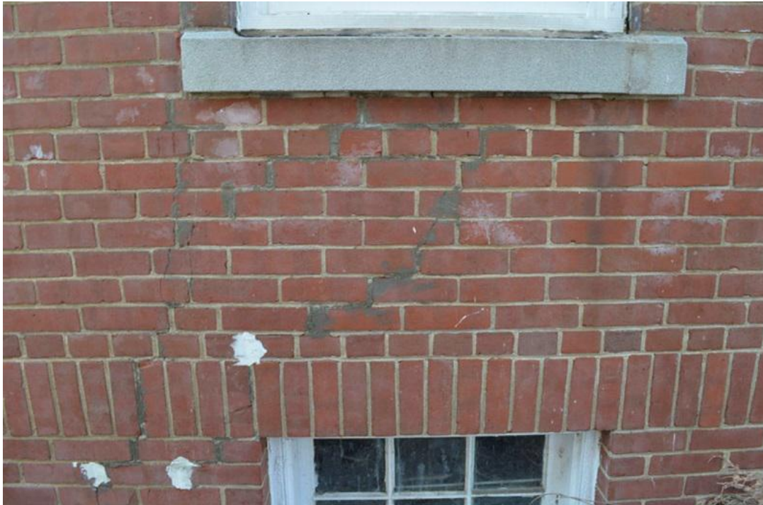
Exterior cracking
