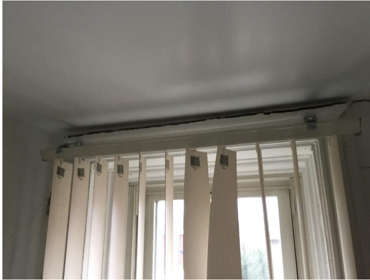
Photo 15: Continuation of cracking noted in photograph 25 above.
