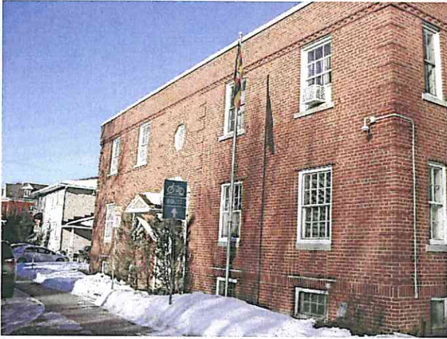
Photo 1 - View of front (west) building elevation.
