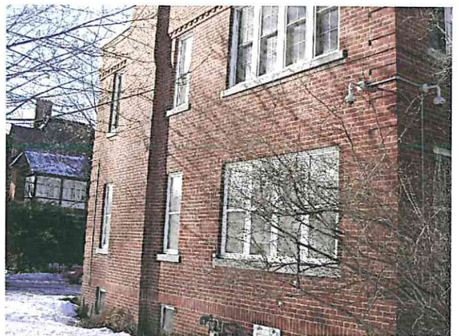
Photo 4 - View of side (south) building elevation.
