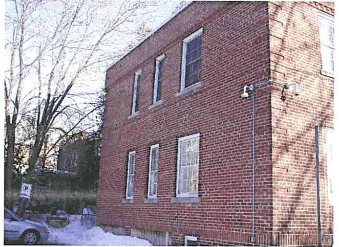
Photo 2 - View of side (north) building elevation.
