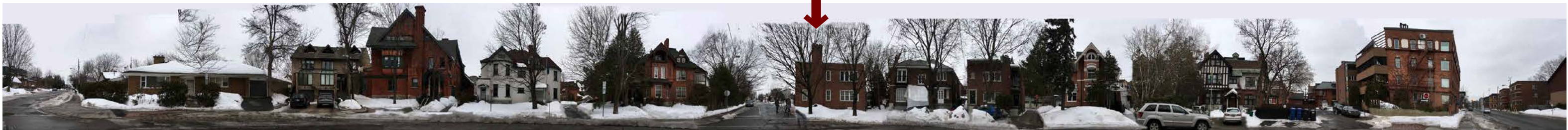
3 EXISTING CONTEXT - Augusta St. To Charlotte St. - North Side A11 SCALE: AS SHOWN
