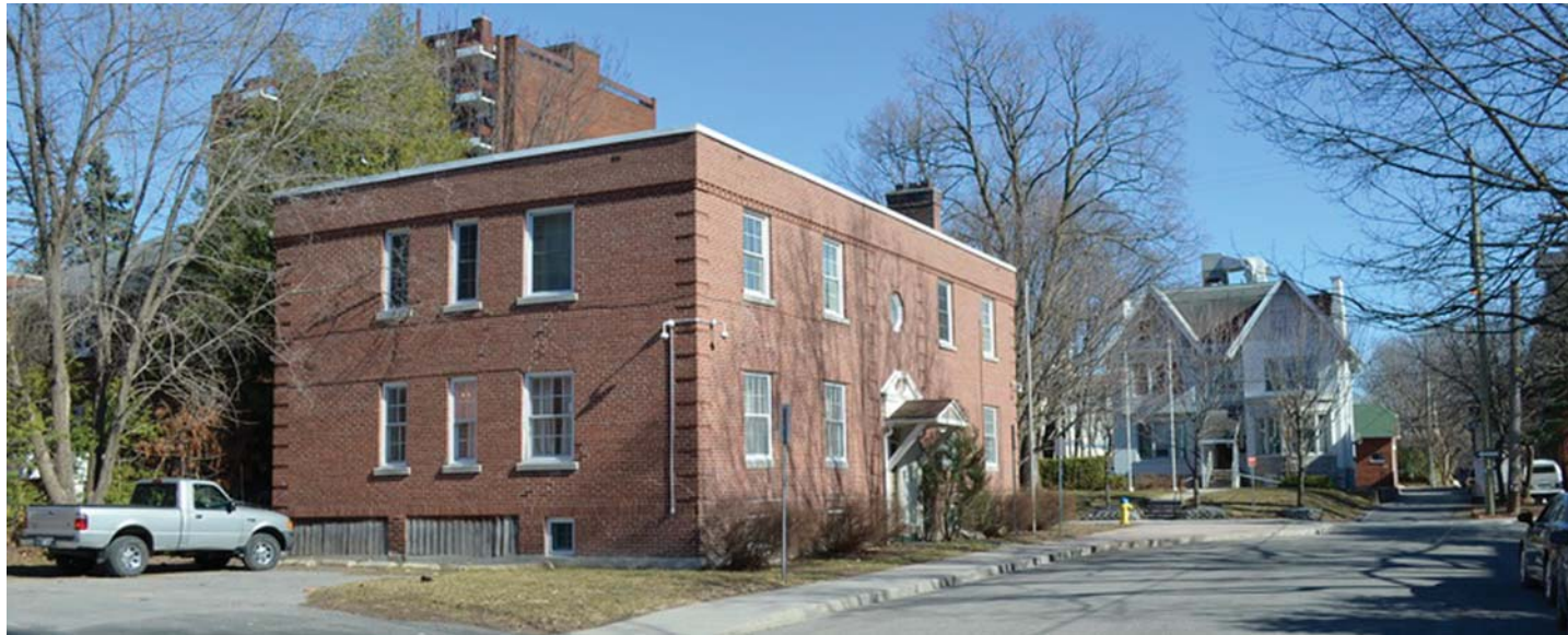
231 Cobourg Street, Ottawa, ON.
