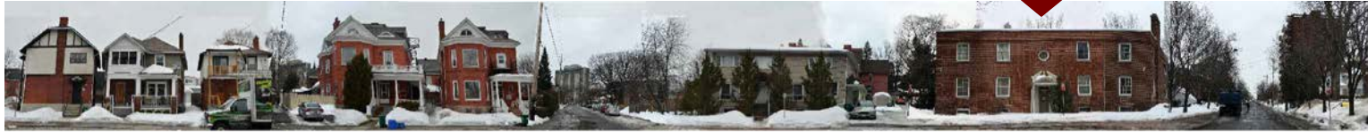
1 EXISTING CONTEXT - Daly Ave. To Wilbrod St.- East Side A11 SCALE: AS SHOWN
