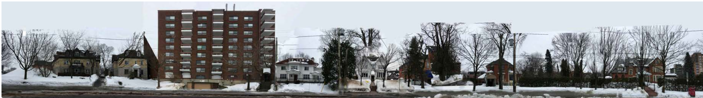
4 EXISTING CONTEXT - Charlotte St. To Augusta St.- South Side A11 SCALE: AS SHOWN
