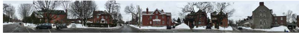
2 EXISTING CONTEXT - Wilbrod St. To Daly Ave. - West Side A11 SCALE: AS SHOWN
