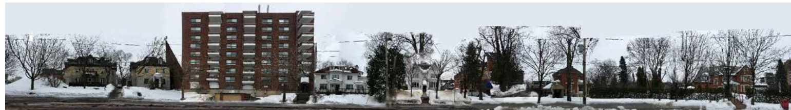
4 EXISTING CONTEXT - Charlotte St. To Augusta St.- South Side A11 SCALE: AS SHOWN
