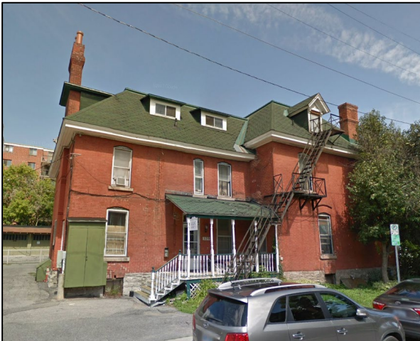
Figure 8: 280 O'Connor Street, side (south) façade of existing building. (Google)
