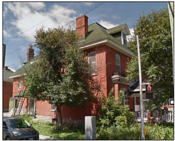
Figure 7: 280 O'Connor Street, corner (south and east) façades of existing building. (Google)
