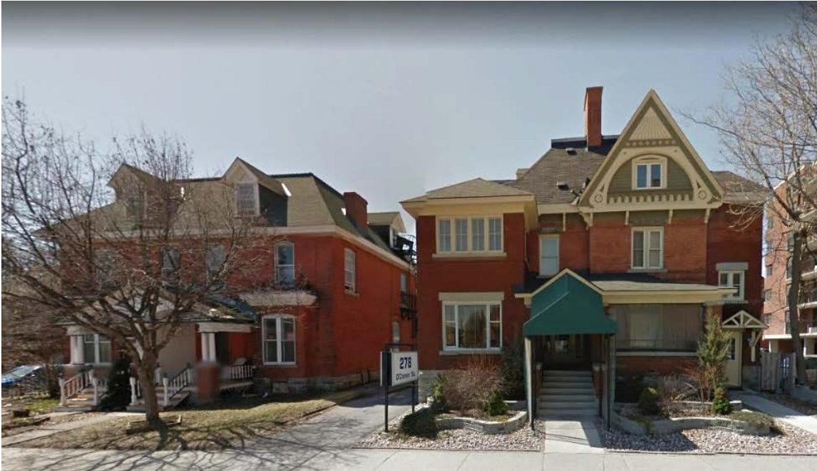
Figure 10: 278 and 280 O'Connor Street (Google May 2016)
