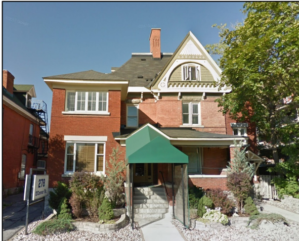
Figure 6: 278 O'Connor Street, front (east) façade of existing building. (Google)
