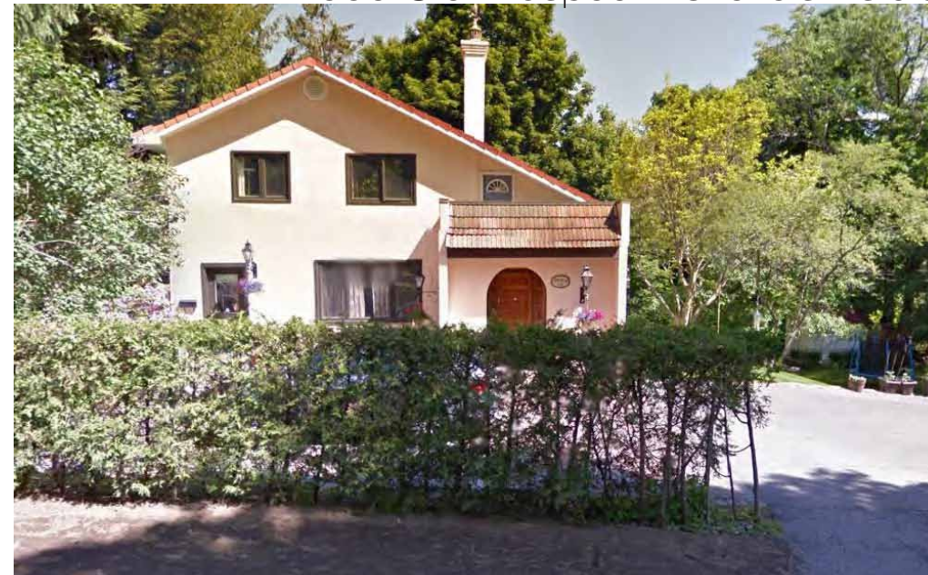
539 Old Prospect - 2 storey
