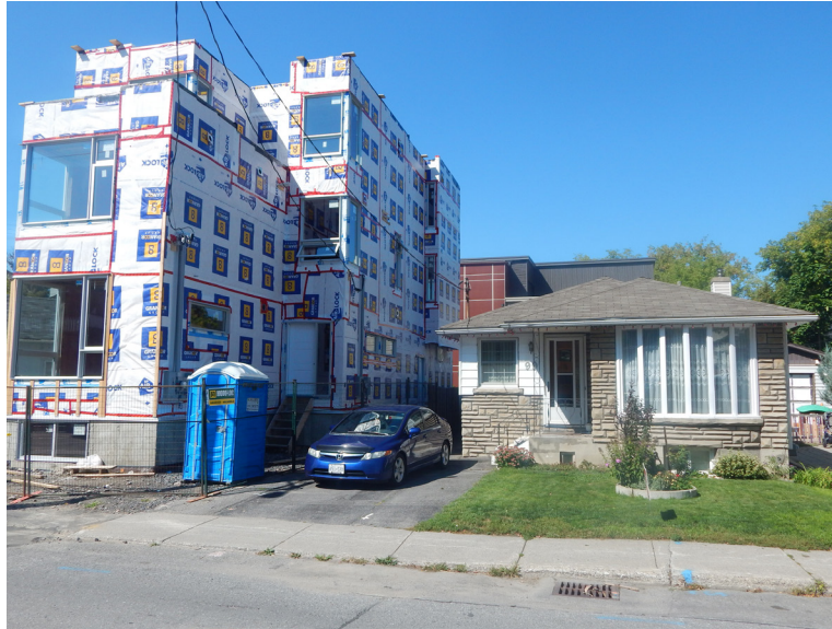
Apartment house in construction on Armstrong Street
