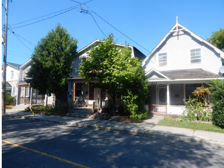
Residential houses on Armstrong Street
