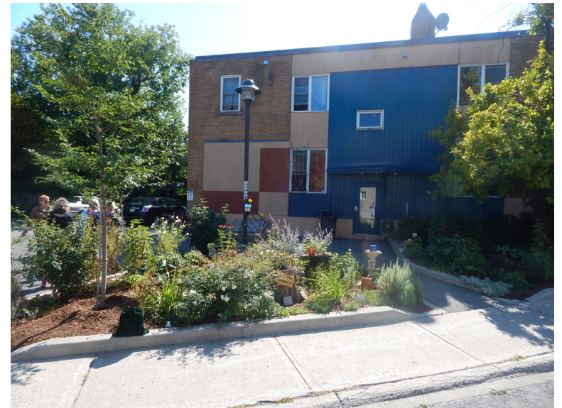
Residential house on Armstrong Street
