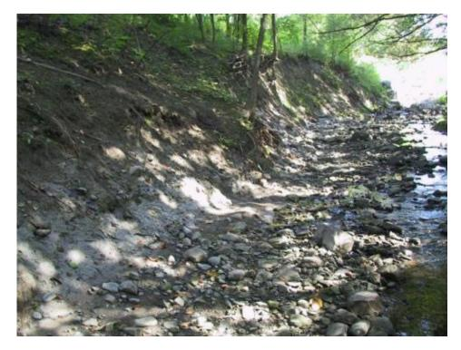
Photo 1: Eroding east bank downstream of gabion wall (Reach 6). View is looking upstream (JFSA, 2015)
