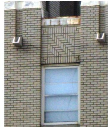
The south and west facades feature less detail than the street facing facades of the building. The geometric panels are not used on the south and west facades, instead the windows have stone sills and brick lintels laid in soldier course. The copper panels are also absent on the south and west facades. The original design of the building and lot included a "parking yard" at the rear of the building.
