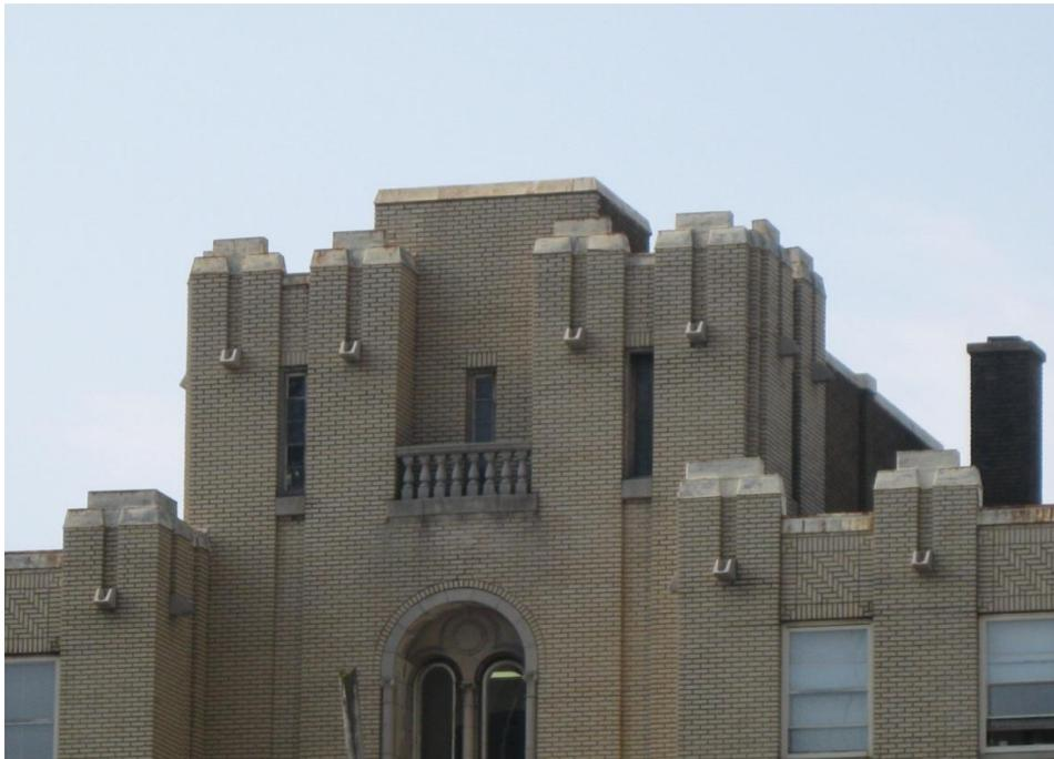
Detailed view of the brick piers that break the roofline and the seventh storey balconet with stone balustrade
