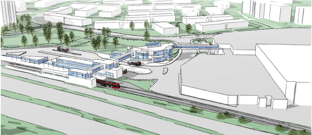
Figure 34: Bird's eye view illustration of Bayshore Station, looking northwest showing LRT and bus platforms and reuse of existing structures
