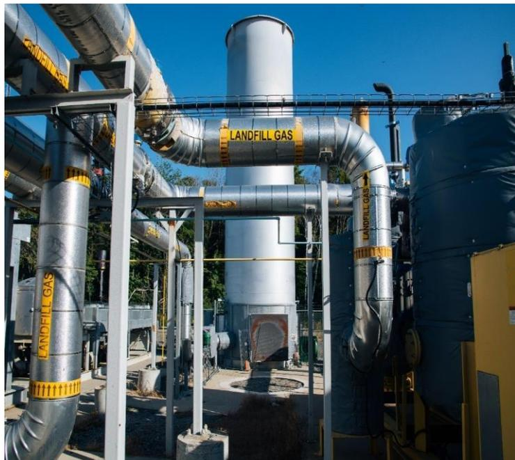
The landfill gas collection system requires expansion as landfilling continues. Following the completion of a landfill section, additional landfill gas collection wells are installed, and the gas collection system is expanded to control odour and allow landfill gas to be collected.
