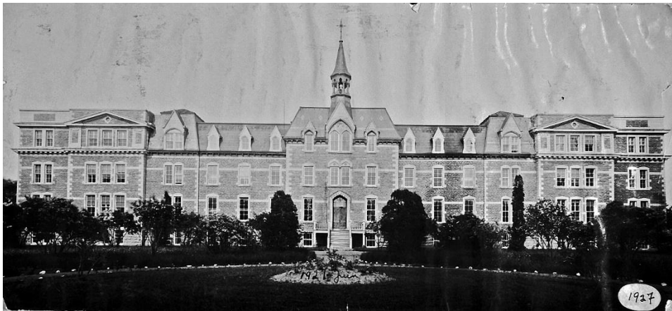
After addition of north and south wings in 1925.
