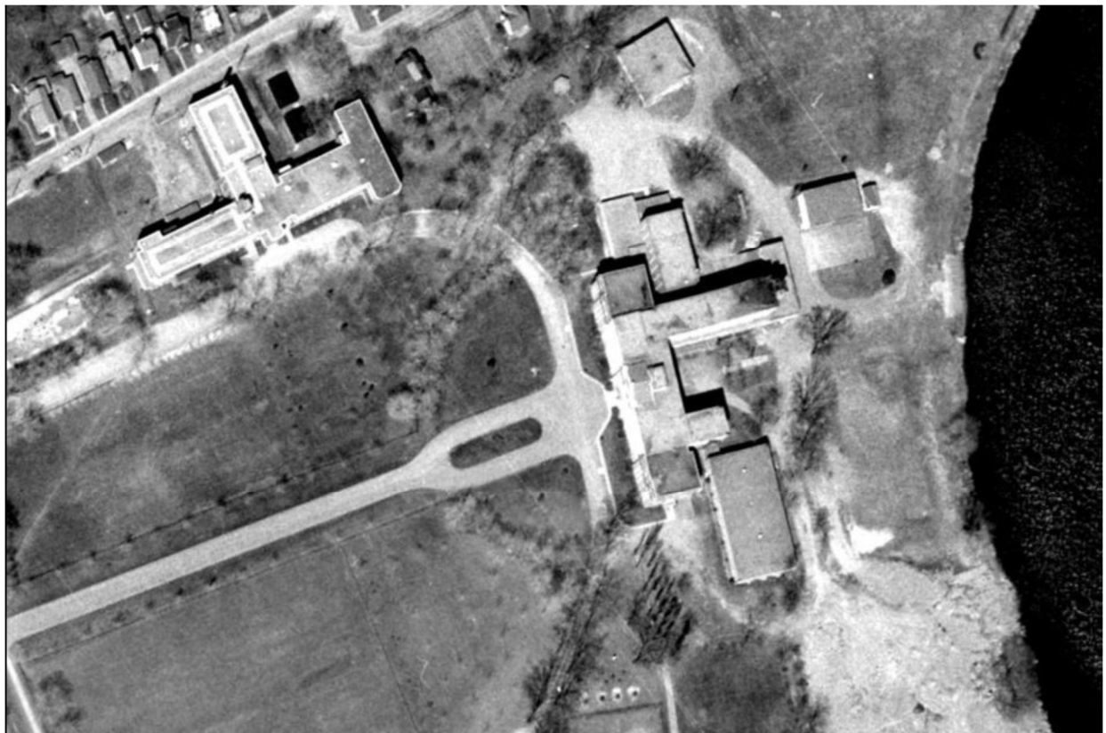
The aerial view of a portion of the Oblate Lands in the late 1960s suggests that the covered veranda has been removed, and the existing verandah is a later addition. The photo is clear, but the south wing is in shadow that may simply be obscuring the roof.
