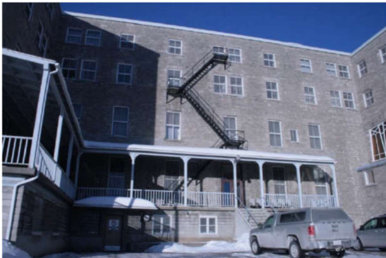
View of veranda along the east elevation with the raised foundation.
