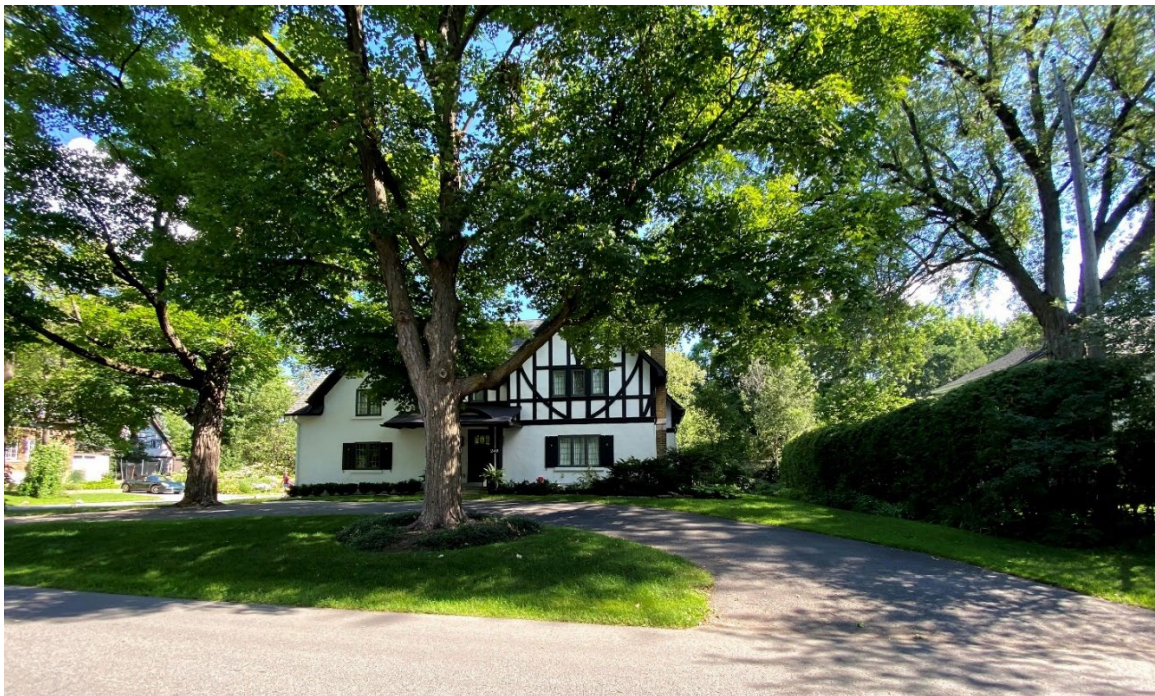
View of house across the street from 235 Mariposa Avenue
