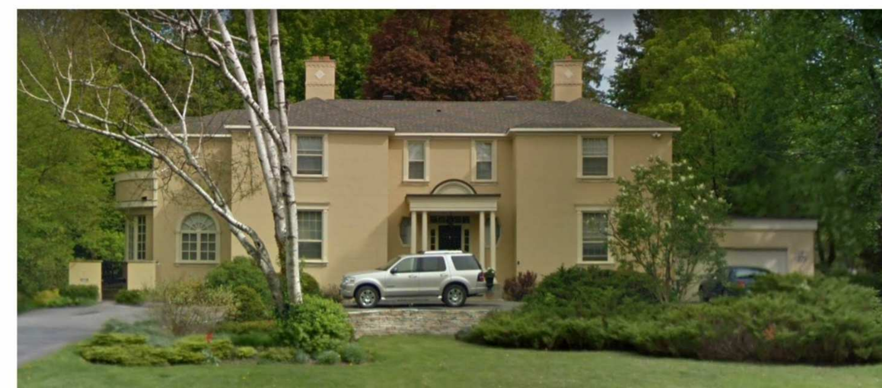
275 Mariposa Avenue Estimated Top of Roof Height: ±9m (based on a visual estimate)
