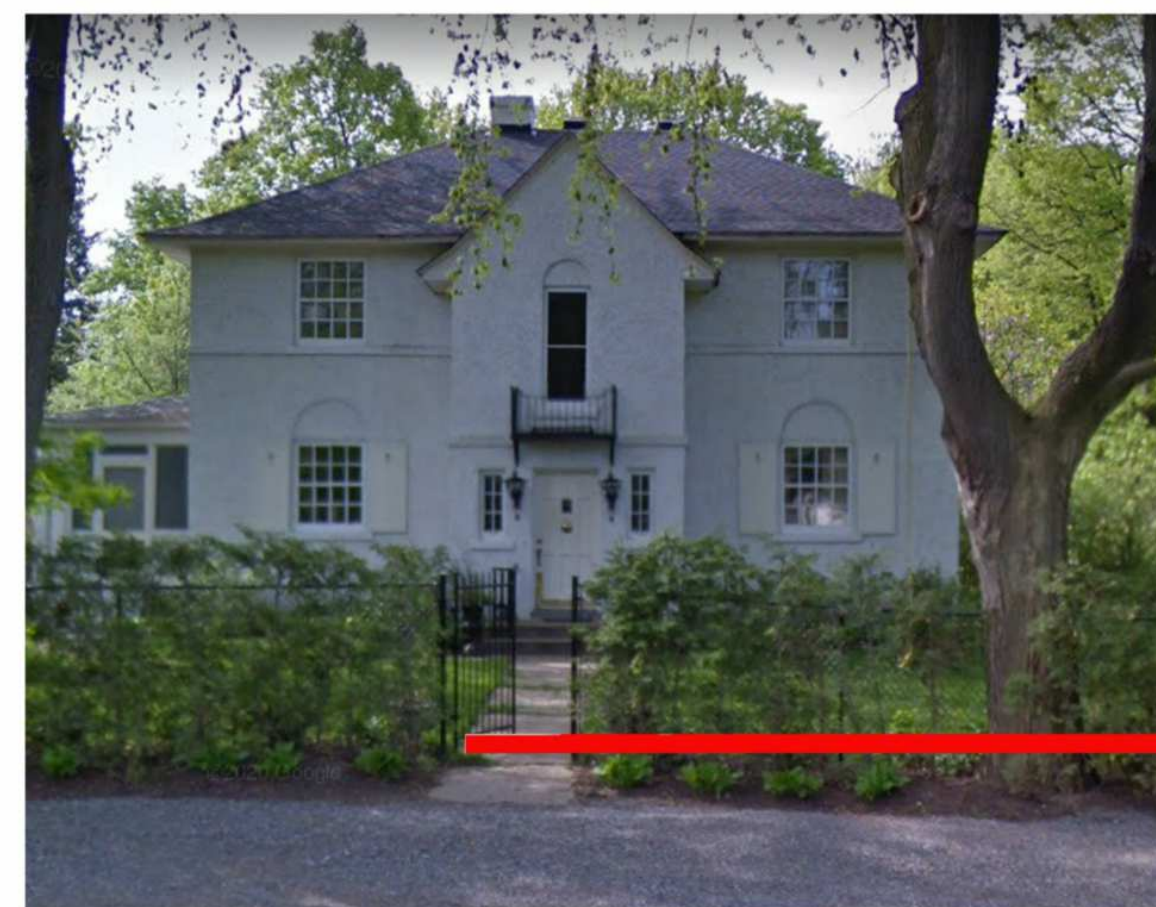
210 Mariposa Avenue Estimated Top of Roof Height: ±12m (based on a visual estimate)
