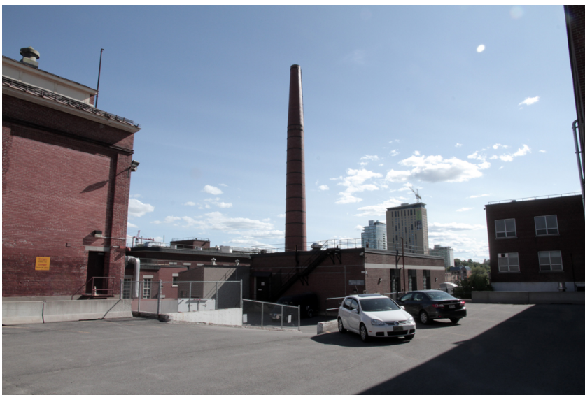
Chimney, Central Heating Plant
