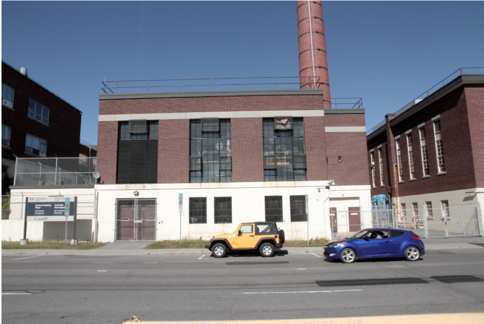
Central Heating Plant
