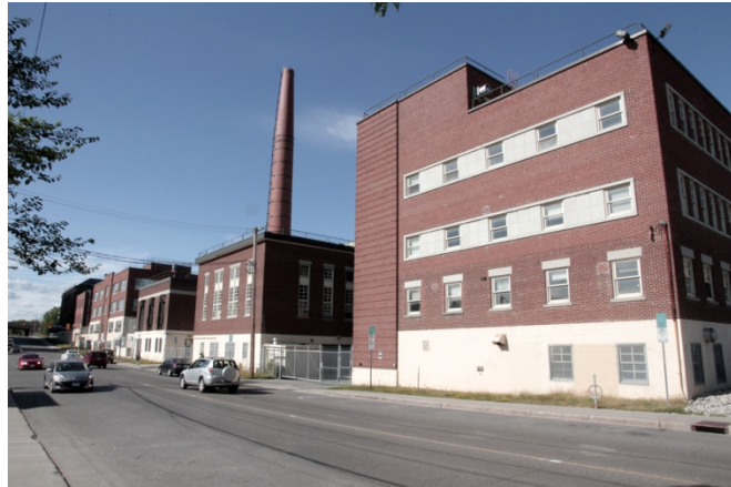
Rear of complex on Rochester Street
